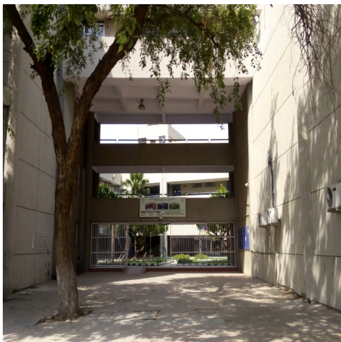
Figure 3.8 Entrance of Civil and Environmental Engineering Department
