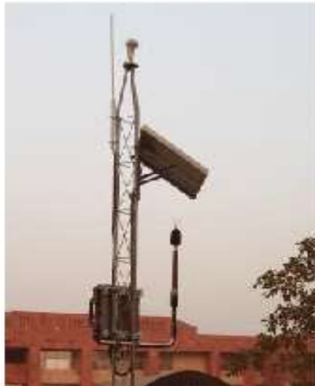
Figure 3.32 Noise level monitoring station installed at DTU.
