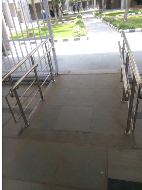
Figure 3.51 Ramp in Electrical Engineering Department
