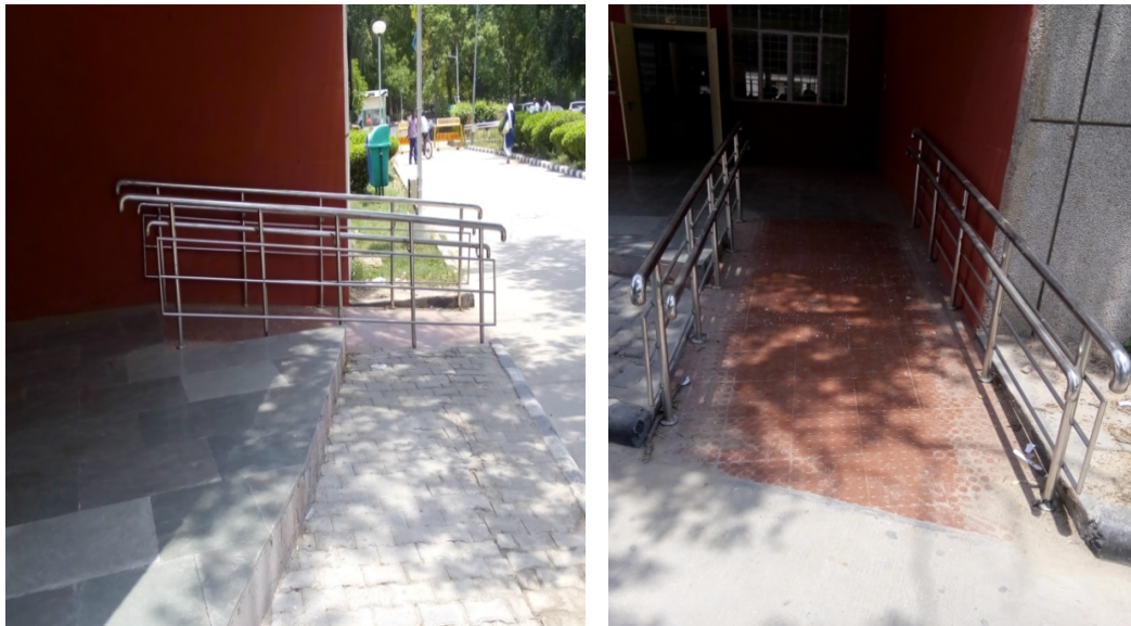
Figure 3.49 Ramps in canteen to make it accessible for physically challenged people
