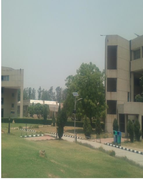
Figure 3.14 Space between Science Block and Mechanical Engineering Block
