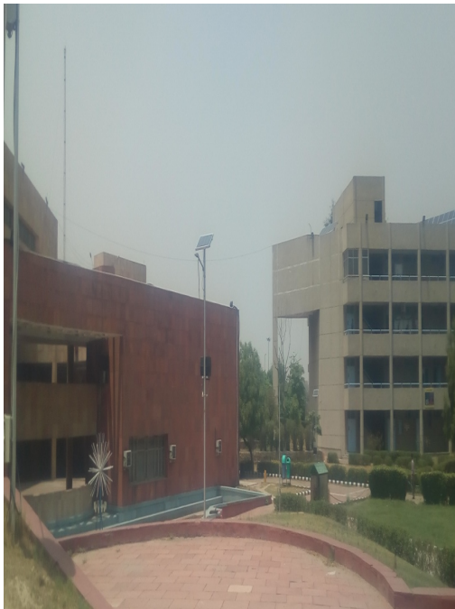
Figure 3.12 Space between Department of Training & Placement Block and Science Block
