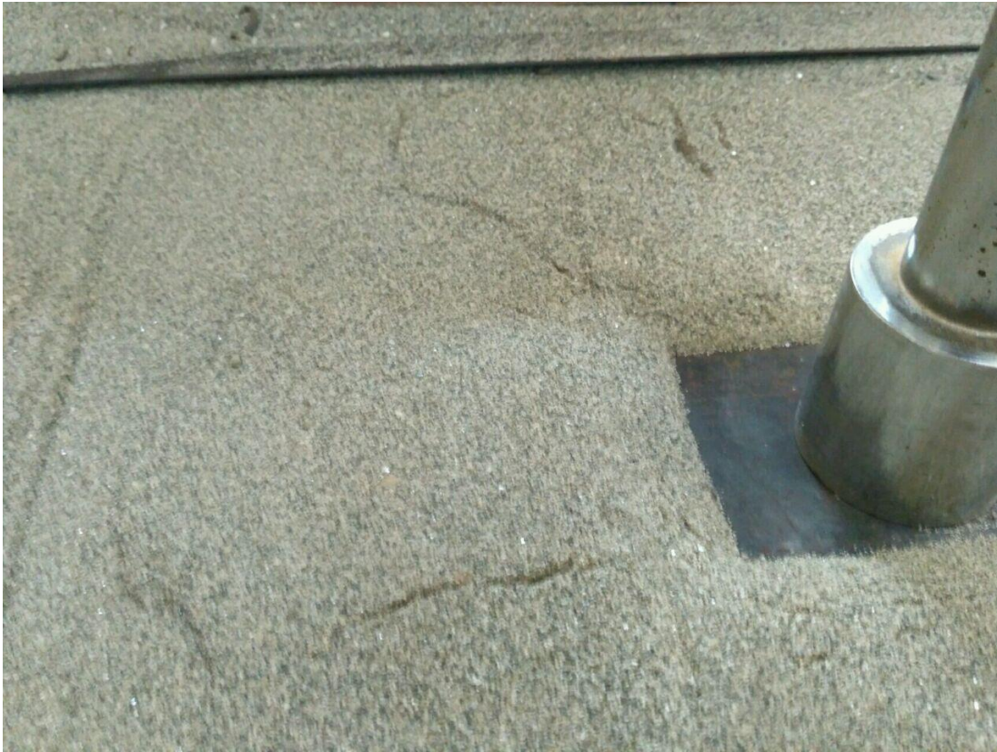
Figure 16 Shear failure of Yamuna sand under 10cmX14cm footing
