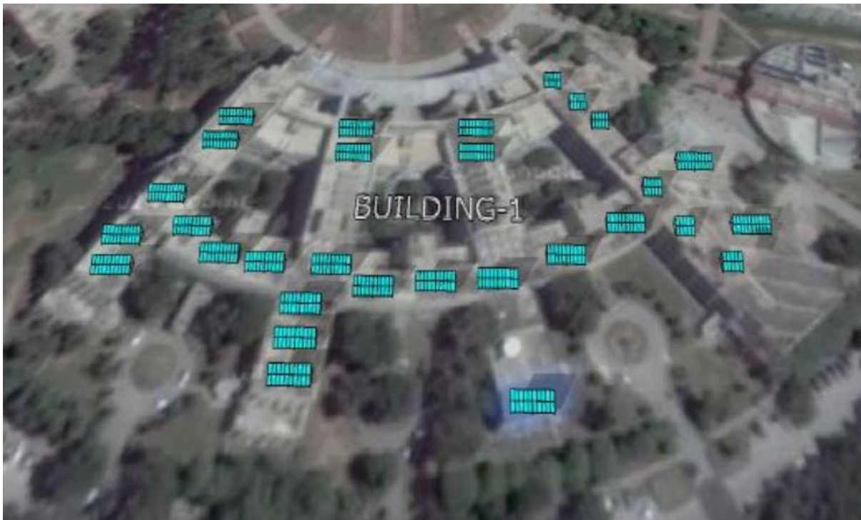
Figure 6.1- View of SPV installed at Building-1
