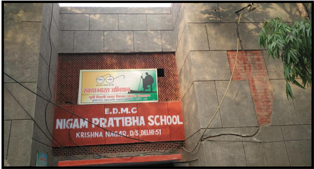
Picture 1: Entrance of school
