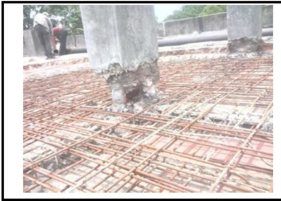
Picture 20: Retrofitting for slab
