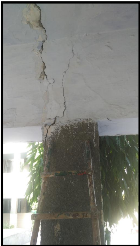
Picture 6: Structural cracks in corridor area of block-C
