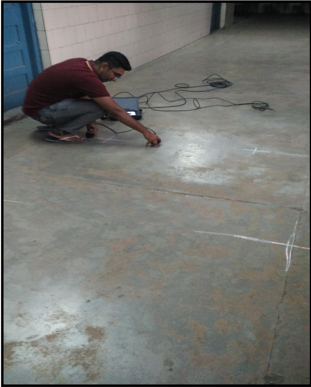
Picture 19: UPVT on slab of block D
