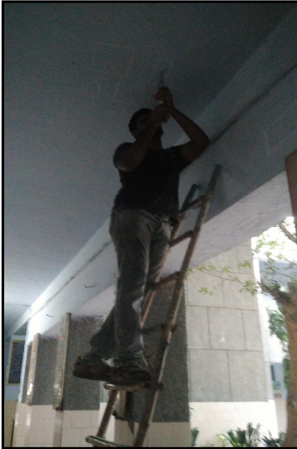
Picture 17: RH Reading on slab of Block A
