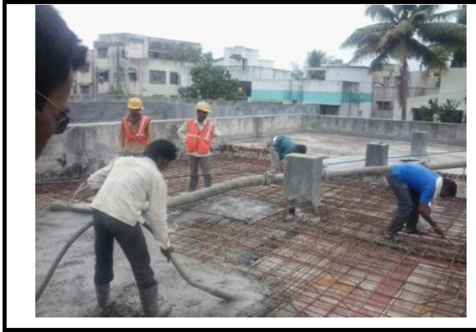
Picture 21: Retrofitting for slab
