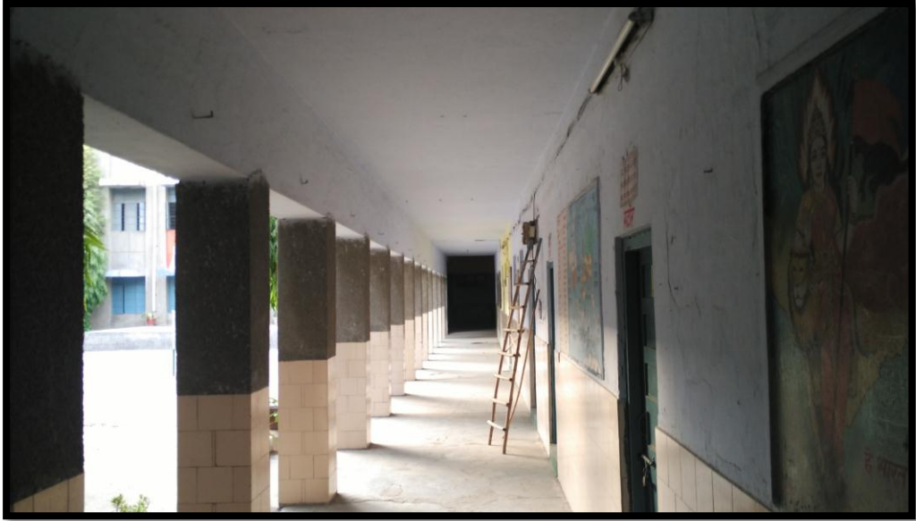
Picture 5: Corridor Area of Block-B
