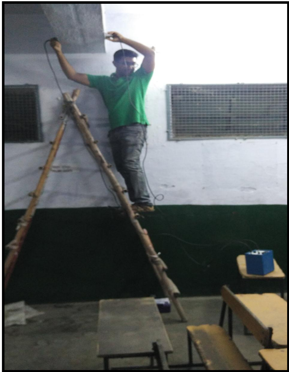
Picture 18: Taking UPVT Reading of beam in block B
