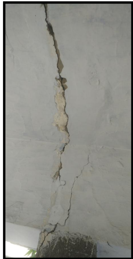
Picture 6: Structural cracks in corridor area of block-C
