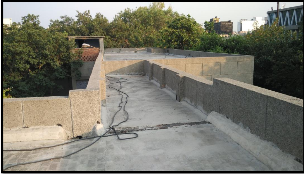
Picture 14: View of Terrace of Block C
