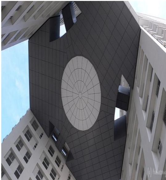
a) Bottom View of sky bridge
