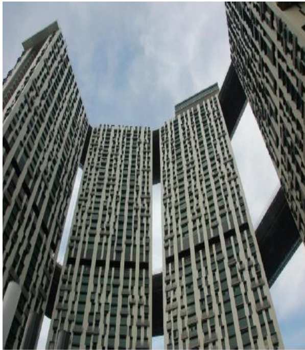
a) Structural View
