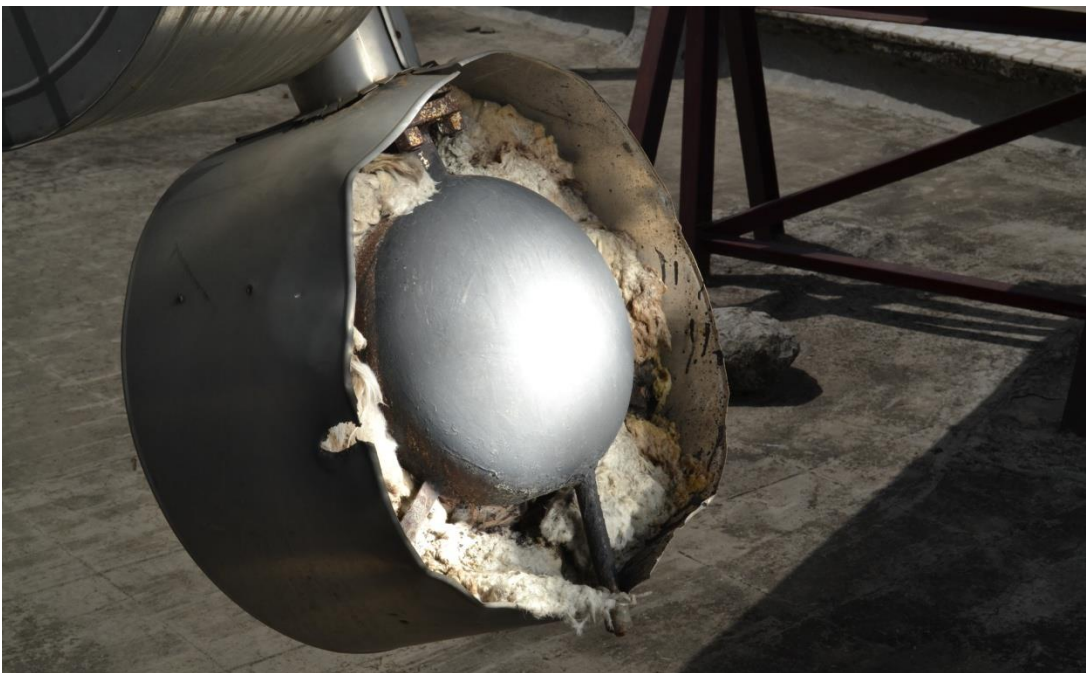
Fig.4.3: Receiver of Scheffler Dish (Drum Type)
