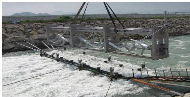
Figure 1.3 Helical turbine instalallation on flowing river in South Korea
