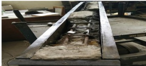
Figure 14: - Fixing beam in the frame
