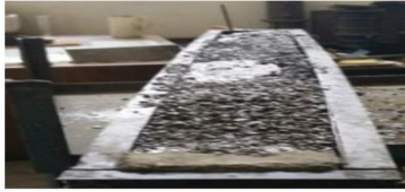
Figure 15: - Pouring of concrete in the frame
