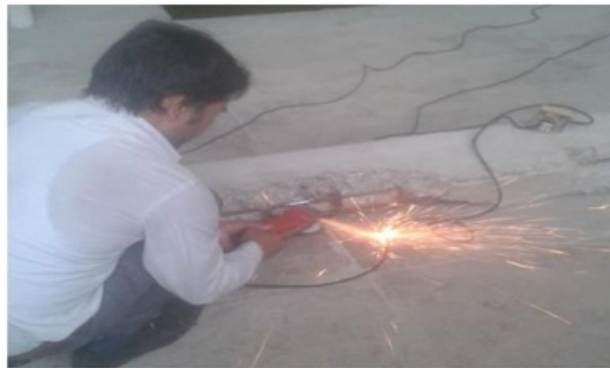
Figure 11: - Grinding of the rebar surface to facilitate fixing of Zinc Anode
