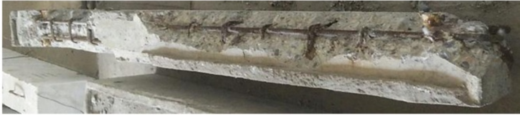
Figure 10: - Beam after removing the defective concrete
