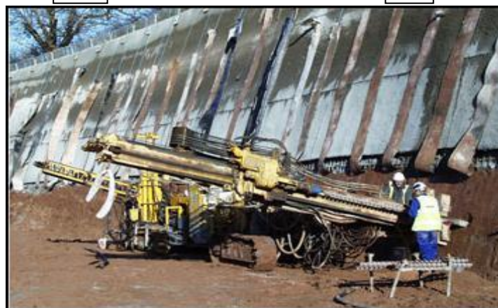
Fig1.1 construction of soil nailed slope (source: http://www.wmplanthire.com/slope_stabilisation.htm )
