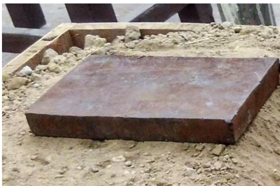
Fig 3.4 Mild Steel Bearing Plate
