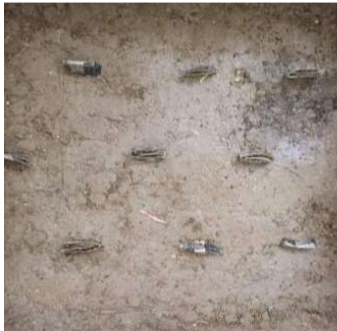
Fig 11 PVDs installed in triangular pattern with s/d=4.0
