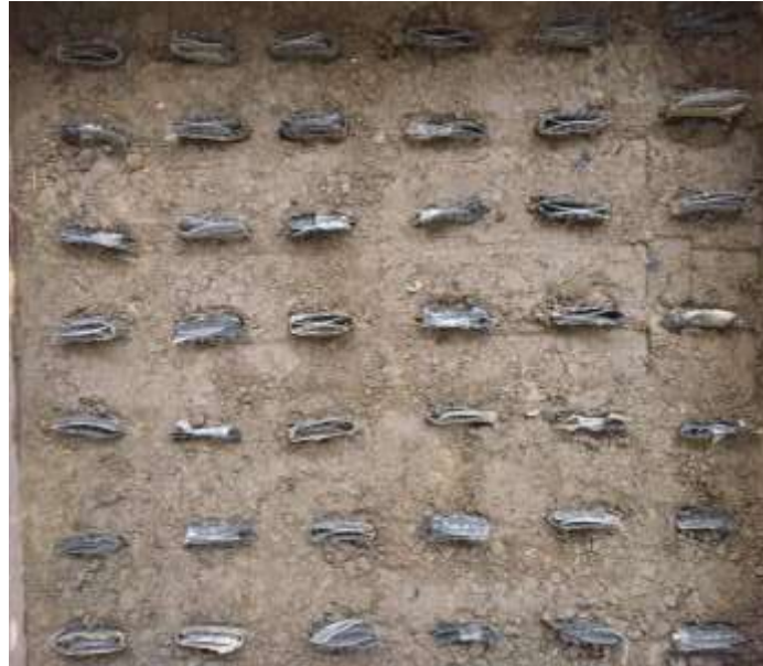
Fig 12 PVDs installed in a rectangular pattern with s/d=2.0
