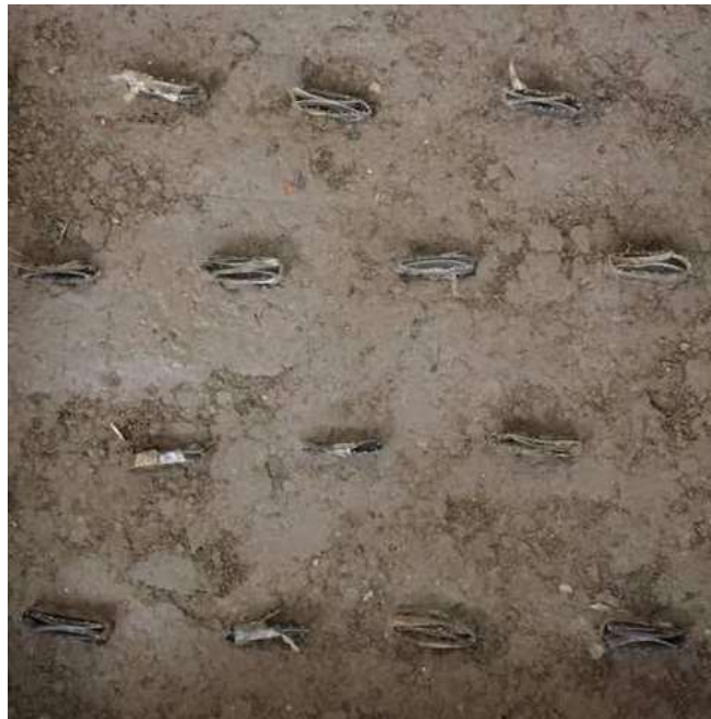
Fig 10 PVDs installed in triangular pattern with s/d=3.0
