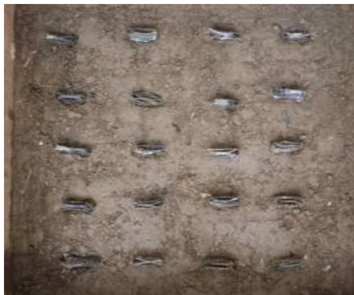
Fig 13 PVDs installed in rectangular pattern with s/d=3.0
