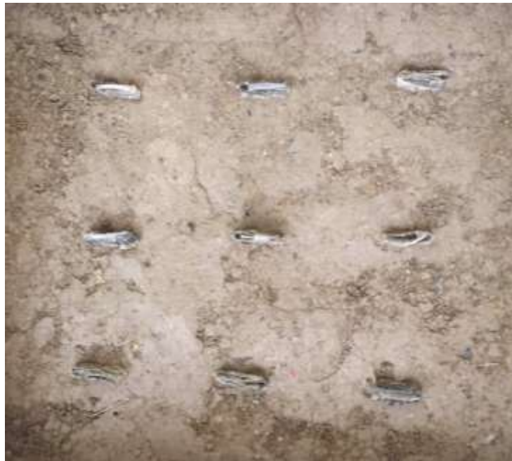
Fig 14 PVDs installed in rectangular pattern with s/d=4.0
