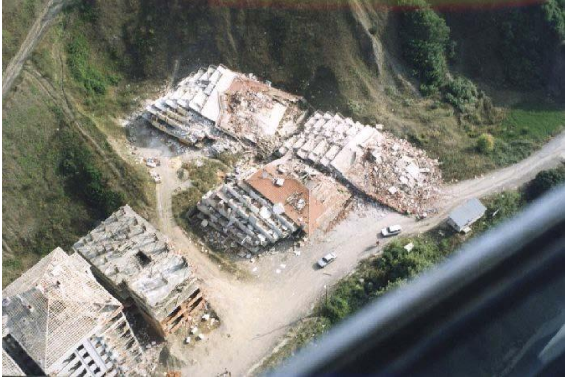
Figure – 2: Collapse of building in earthquake
