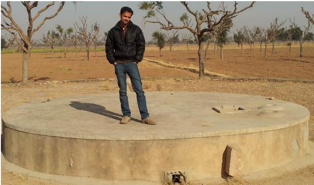
Figure 2.7: Rainwater harvesting tank (popularly called taanka ) on a road side in one of the fluoride hit area of Rajasthan
