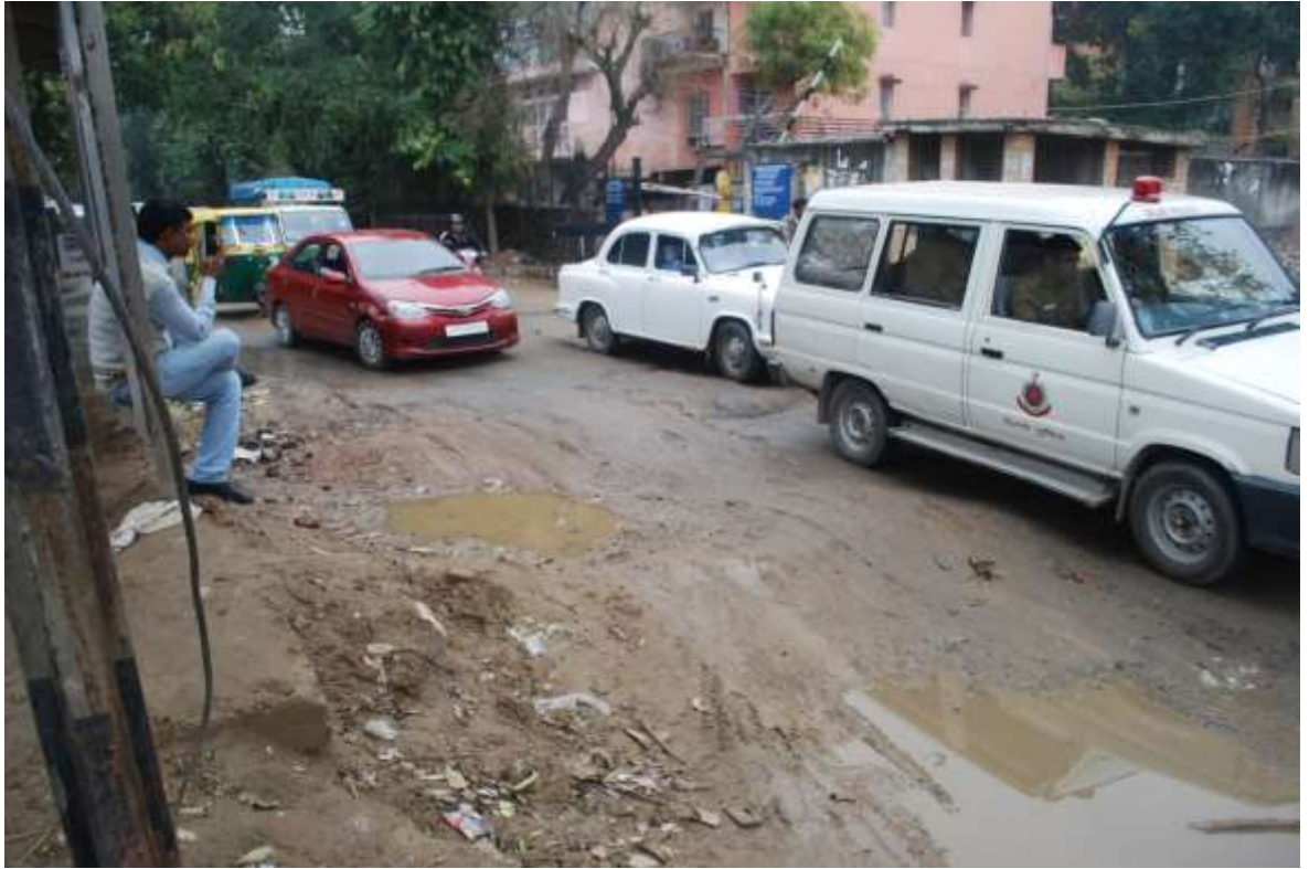
Figure 4: Damaged existing road , no proper drainage system
