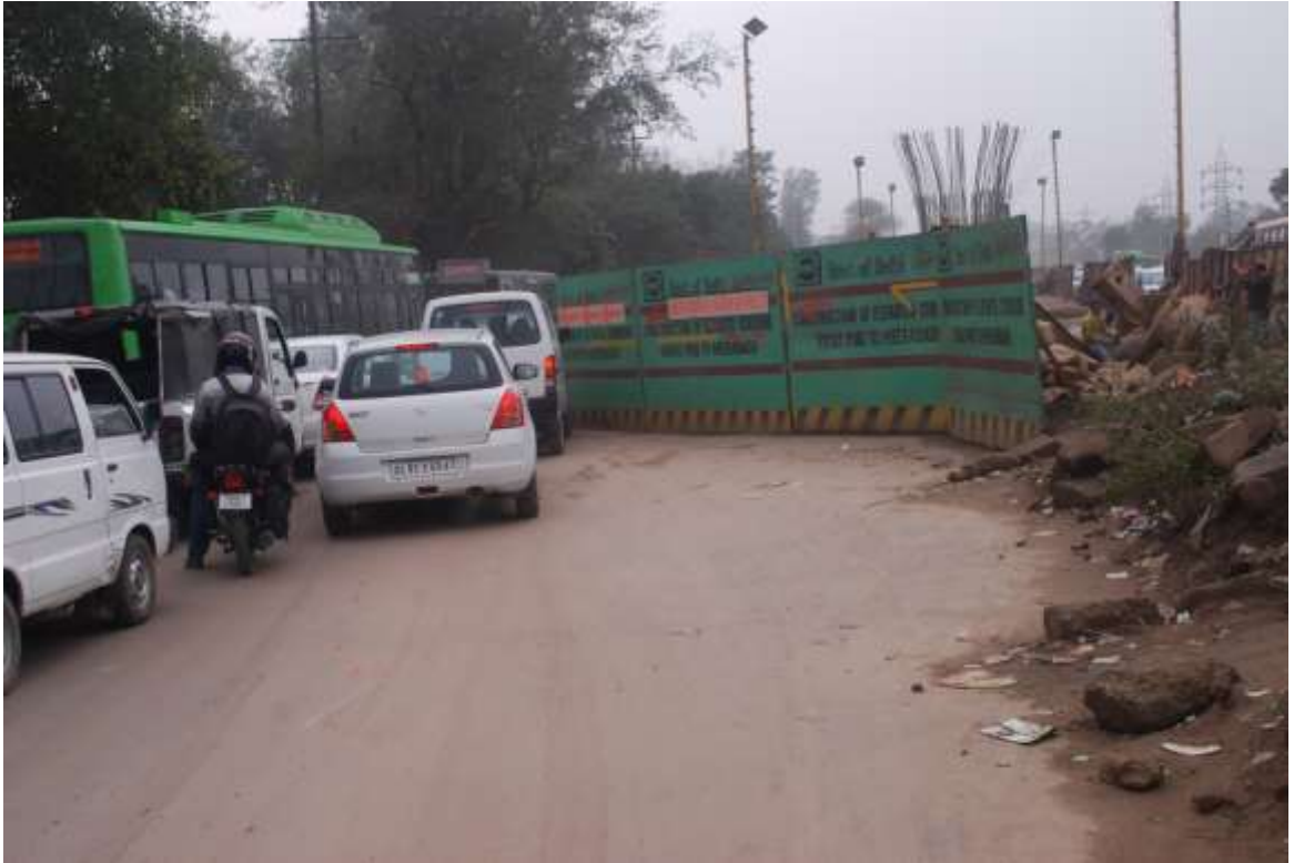
Figure 3: Improper, merging and porous barricades causing traffic congestion, Jam, more fuel consumption, CO 2 emission.
