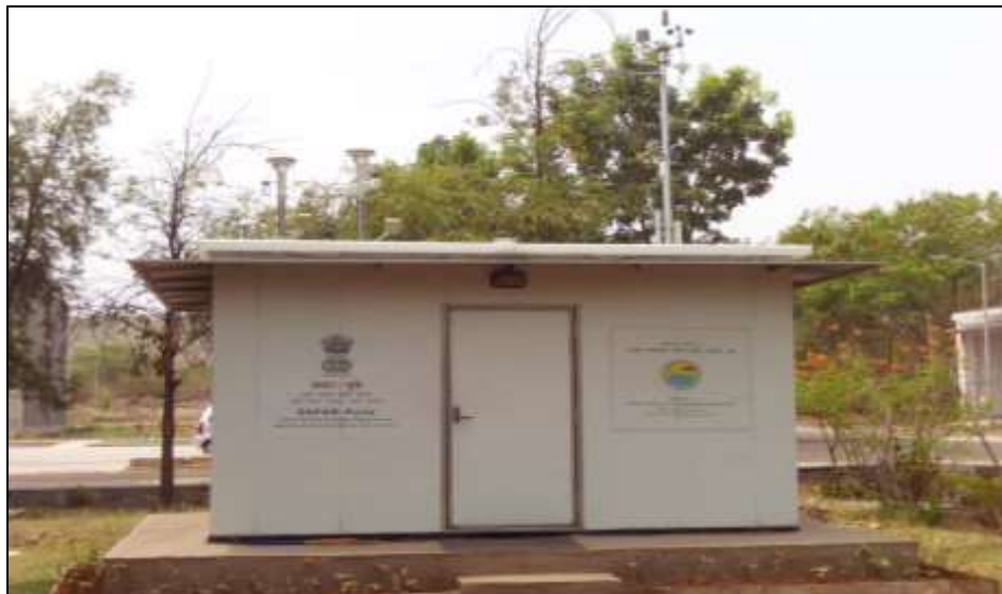
Figure 3.1 – Actual Site of Monitoring Station of IITM
