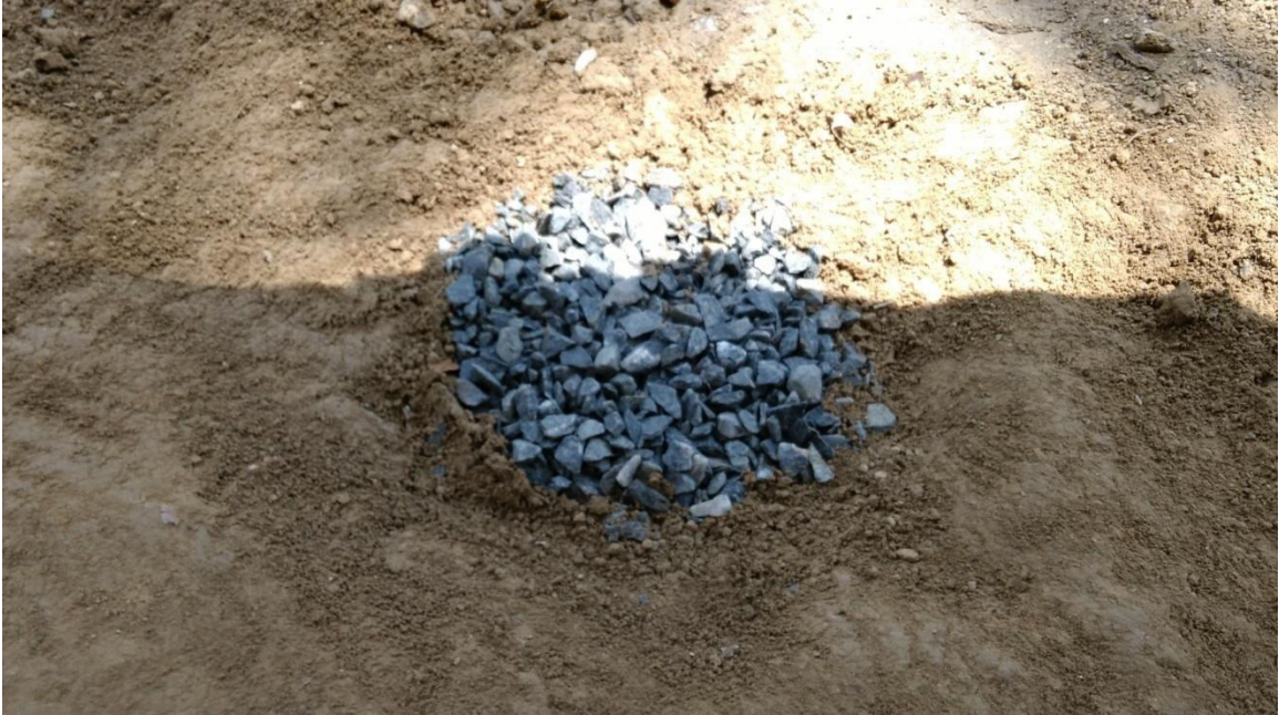
Fig. 4.3 Stone column after complete withdrawn of PVC pipe
