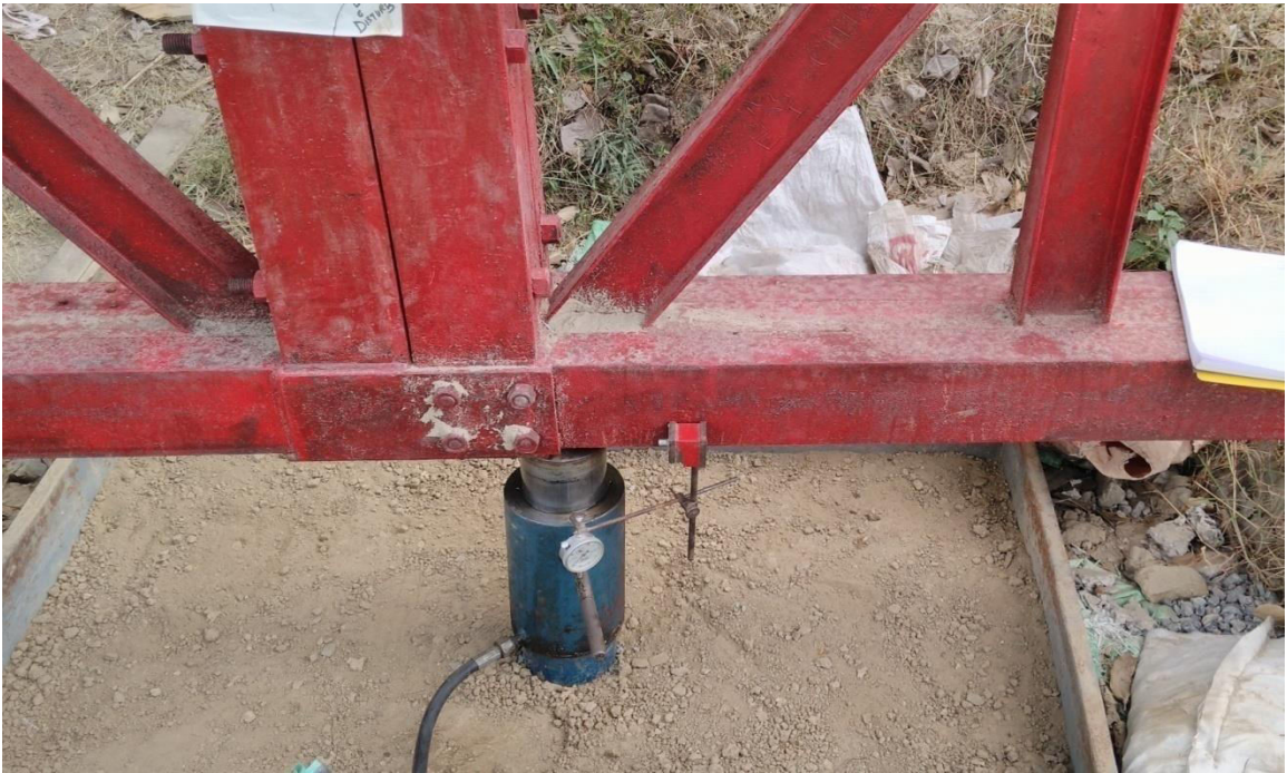
Fig. 4.4 Load applying by Hydraulic jack on stone column
