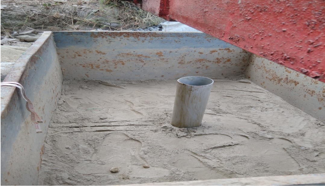
Fig. 4.1 Placing of PVC pipe at the location of stone column
