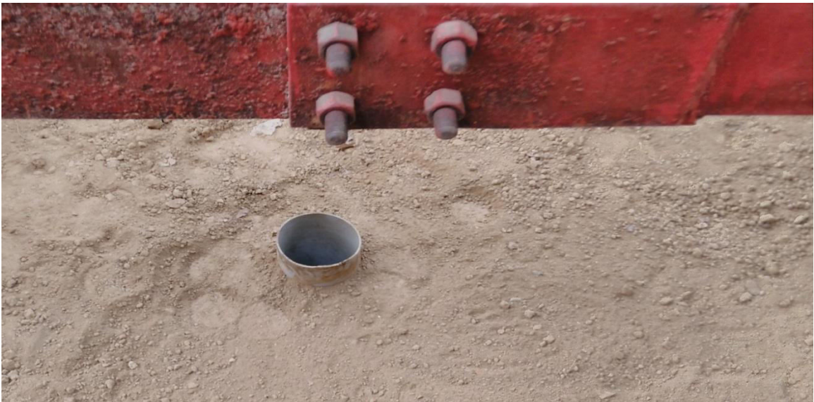
Fig. 4.2 Soil filling up to design level in tank
