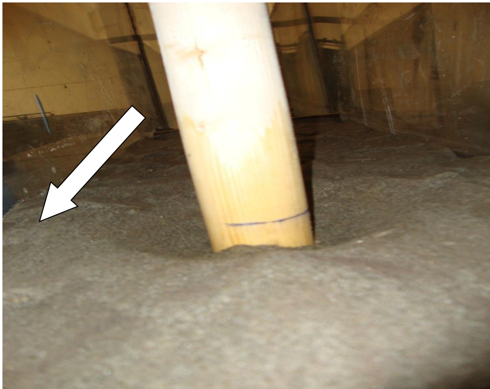
Figure: 5.6 Scour around cylindrical pier at downstream side
