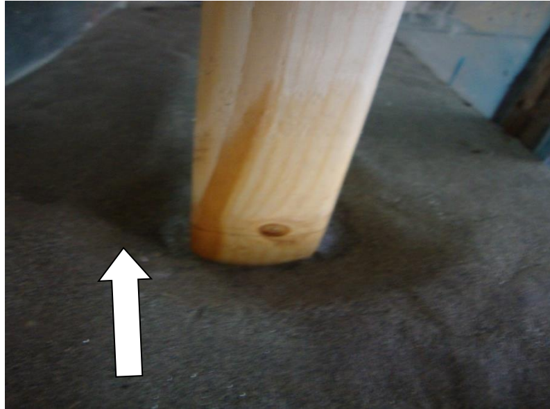
Figure: 5.7 Scour around round-nose pier at upstream side along the channel flow( \Theta=0^0 )
