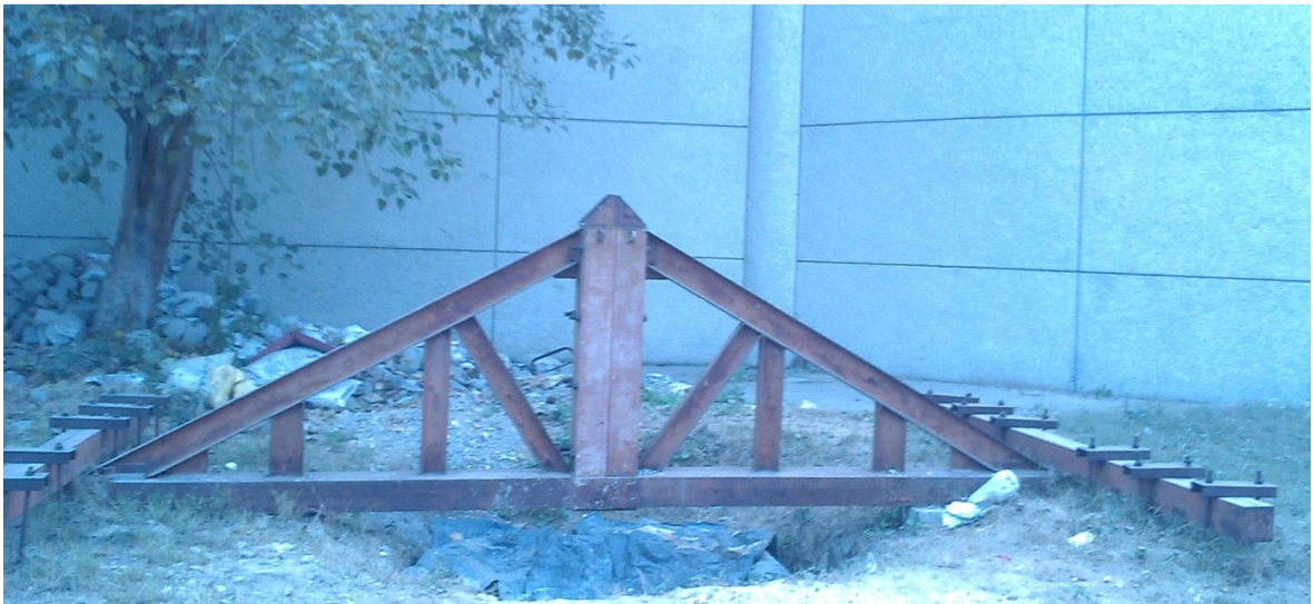
Picture 2: Truss used for loading
