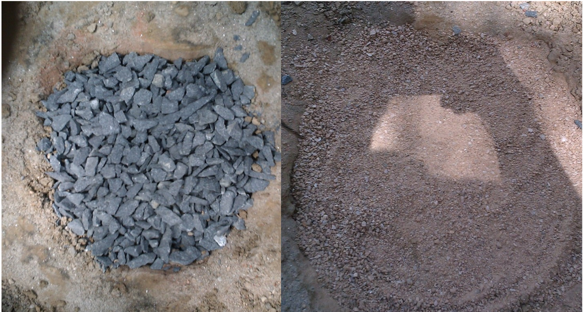
Picture 12: Stone column with 10mm aggregate and sand layer on top of stone column
