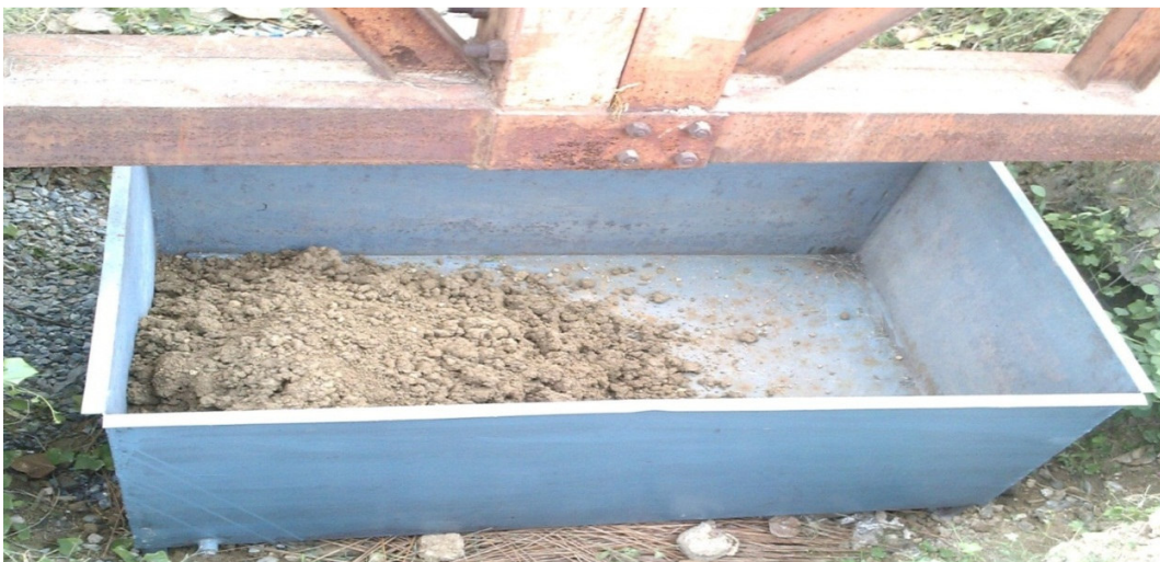
Picture 5: Rectangular tank soil filling (1.5m×0.6m×0.9m)
