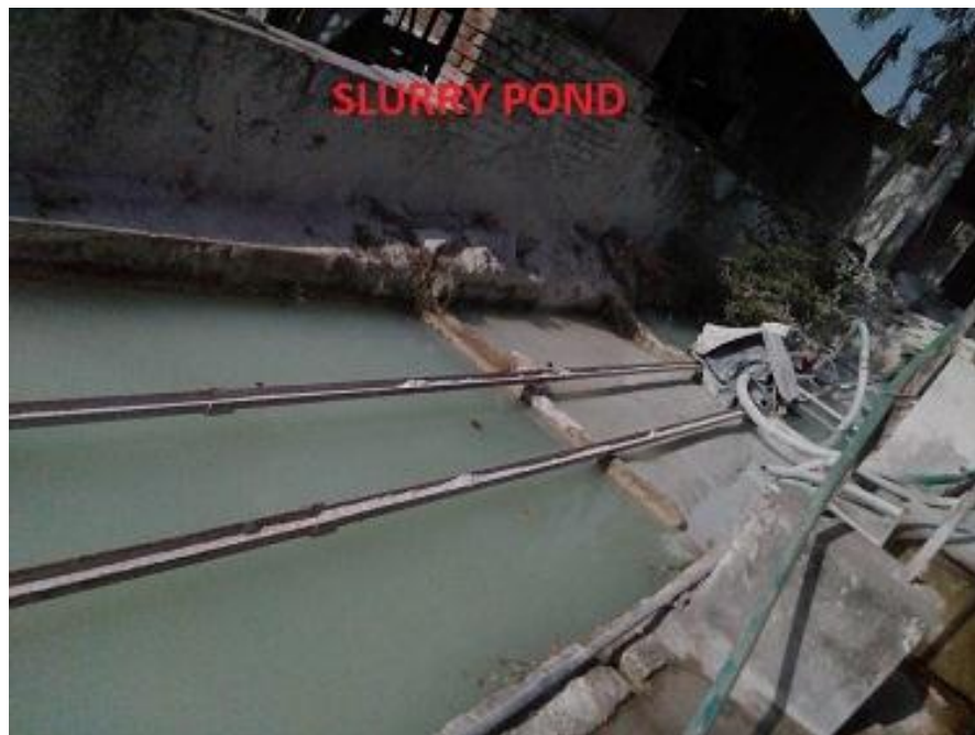
Figure 1.2: Slurry Pond to Settle Stone Dust
