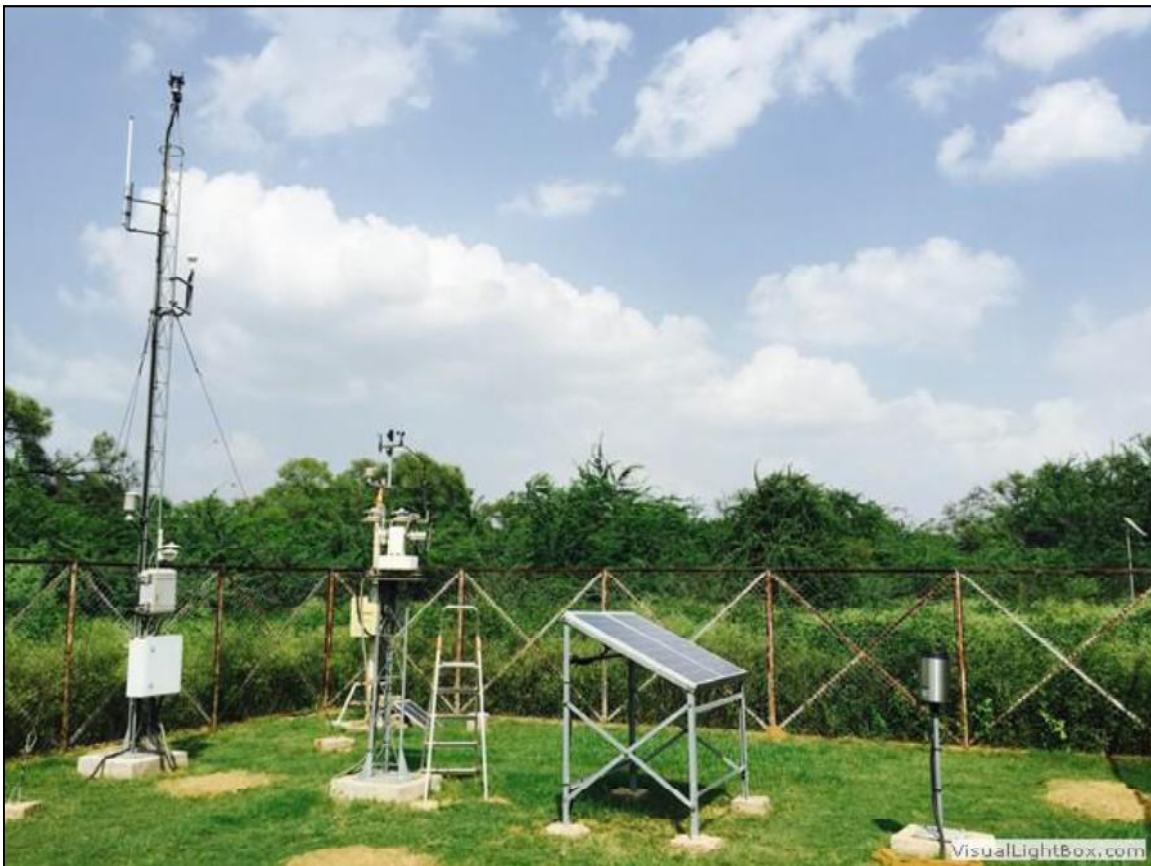
Figure: 3.1, a typical Solar Radiation Resource Assessment (SRRRA) Station [49]
