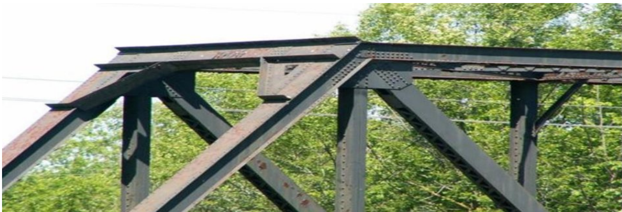
Fig. 2.10 portal bracing
