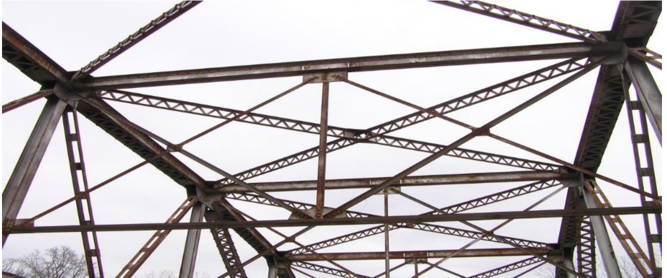
Fig. 2.9 sway bracing
