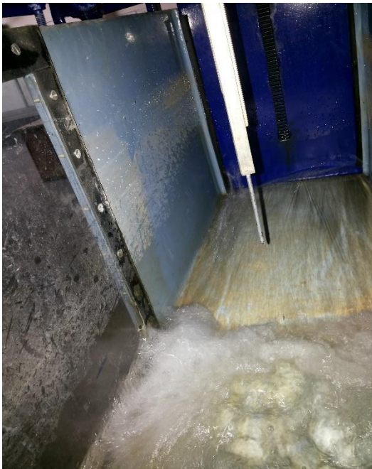
Figure 14: Hydraulic Jump from the Sluice Gate
