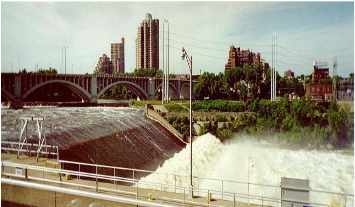
Figure: 1.1 Condition of formation Hydraulic jump (Saint Anthony Falls in Minneapolis)
