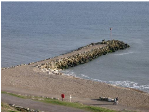
Fig. 1.2. Impermeable Groyne
