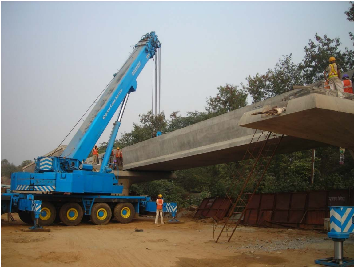
Figure 3.23 Erection of U - Girders
