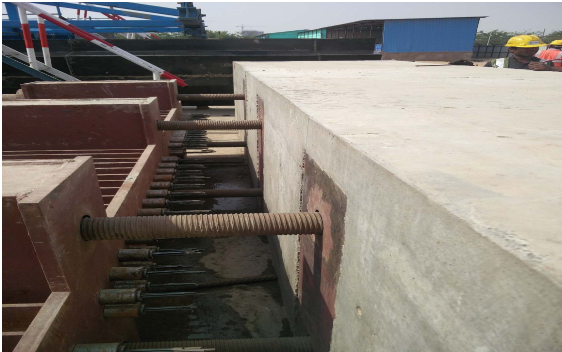
Figure 3.16 Strands Anchored with Wedges at Prestressing End
