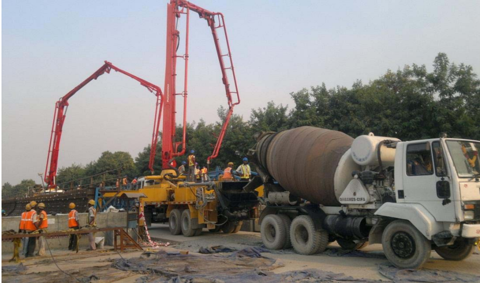
Figure 3.18 Casting of U – Girders
