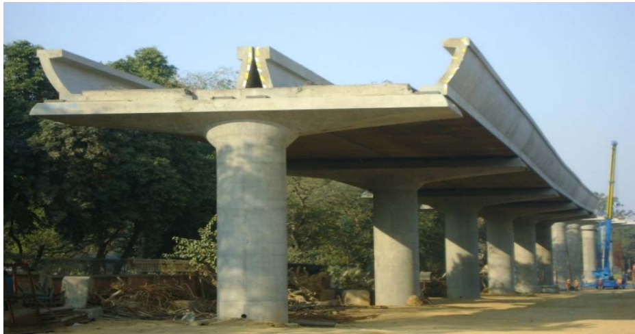
Figure 1.1 A Typical Twin U – Girder Viaduct
