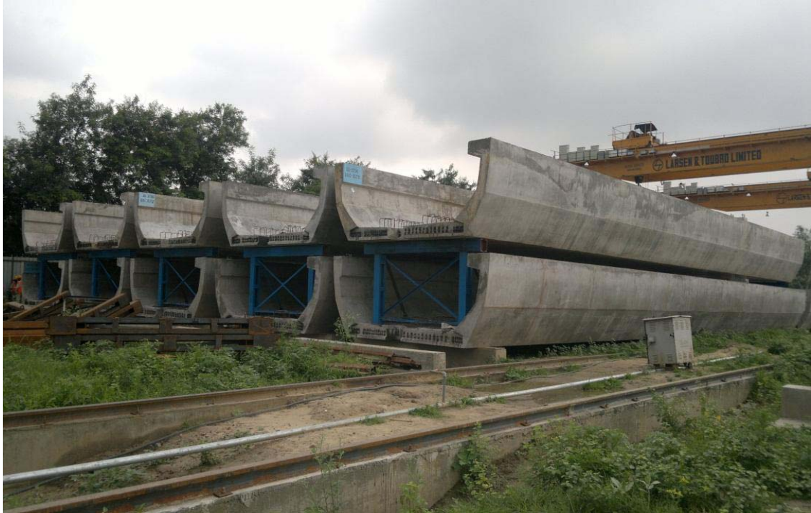
Figure 3.21 Stacking of Casted U - Girders
