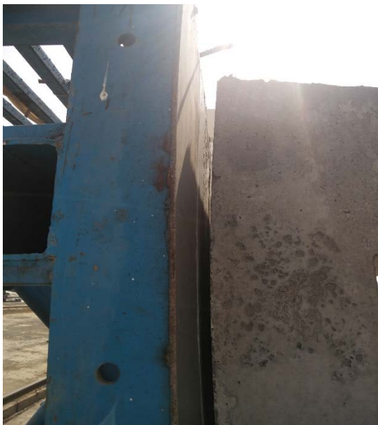
Figure 3.19 Removal of Formwork
