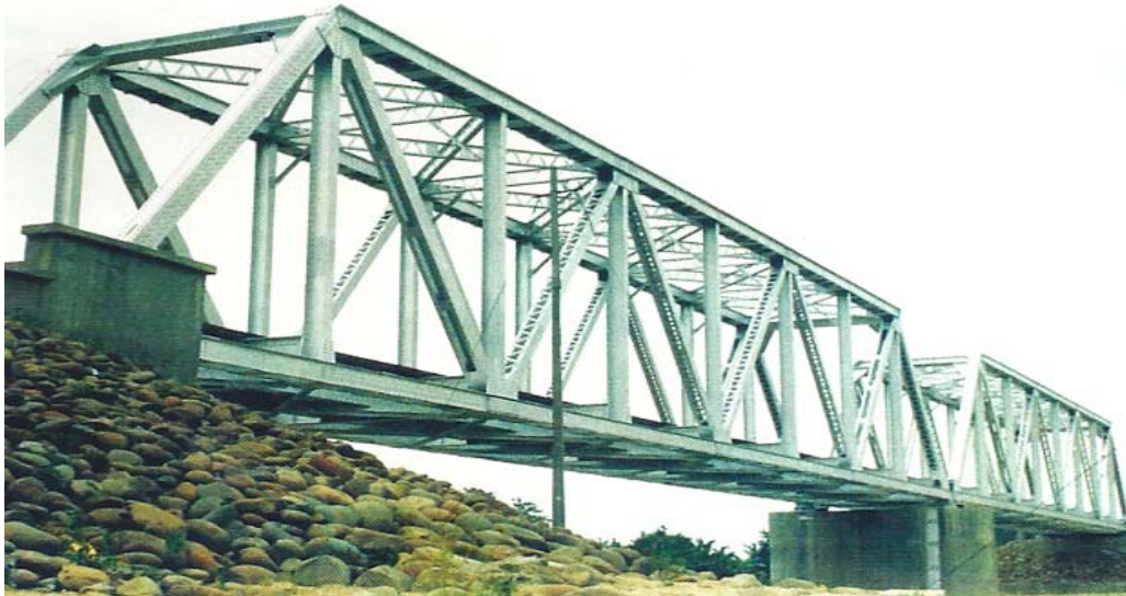
Figure 3.3 A Typical Through Type Bridge
