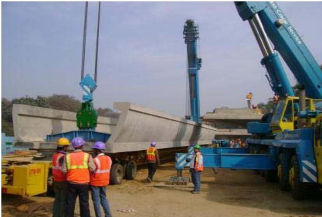
Figure 3.22 Loading and Unloading of U - Girders
