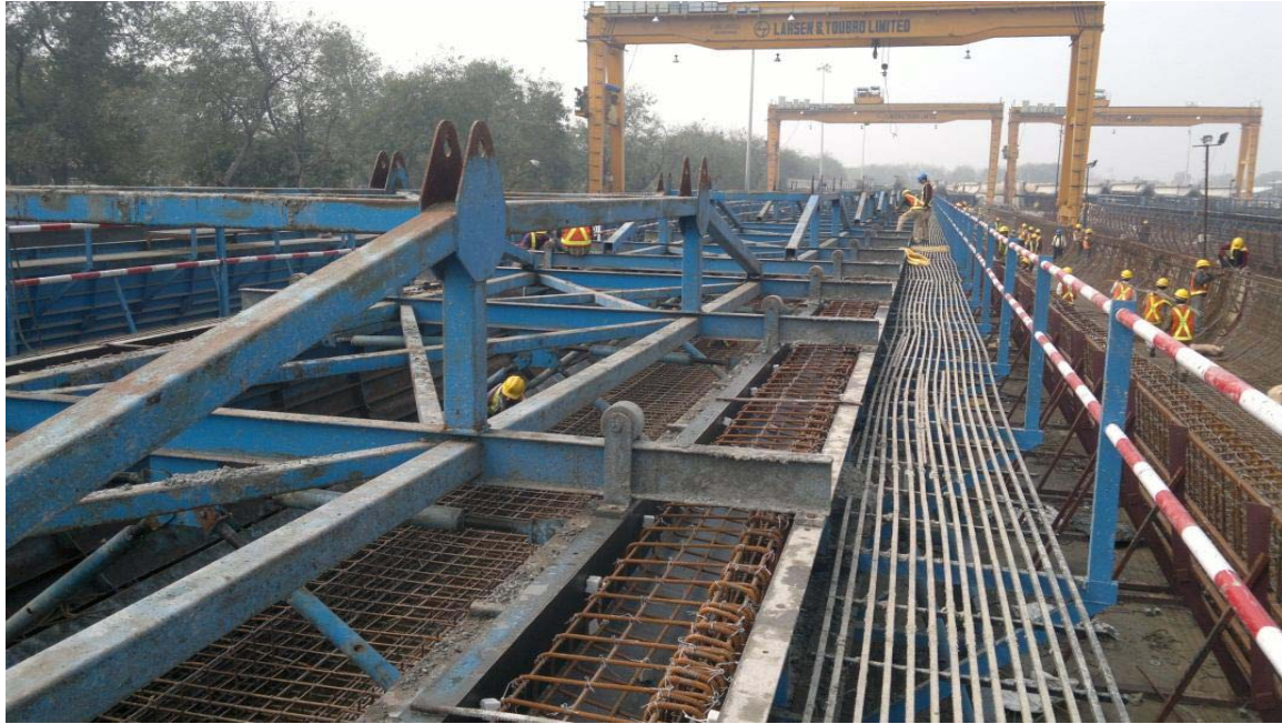
Figure 3.12 Installation of Formwork for Inside Surface of U-Girder
