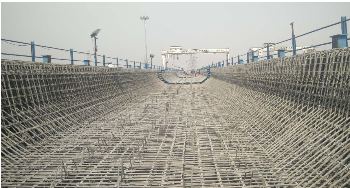
Figure 3.11 Placement of Reinforcement Cage in the Prepared Formwork
