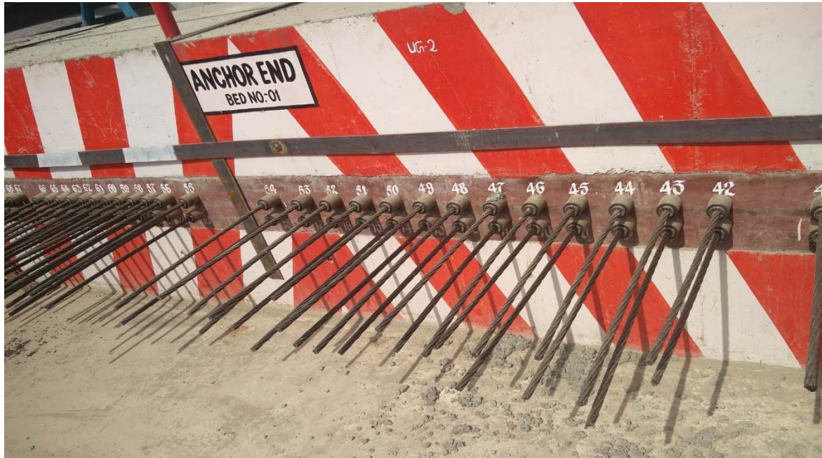
Figure 3.14 Strands Anchored with Wedges at Anchor End
