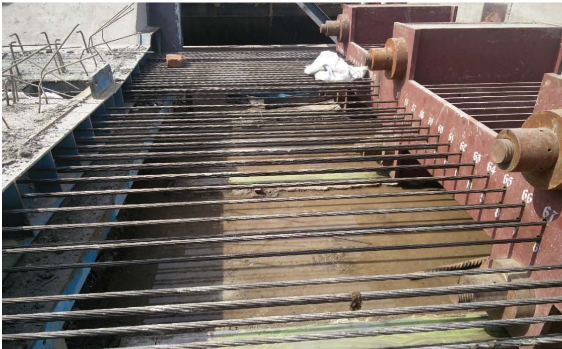
Figure 3.15 Prestressing of Strands at Prestressing End
