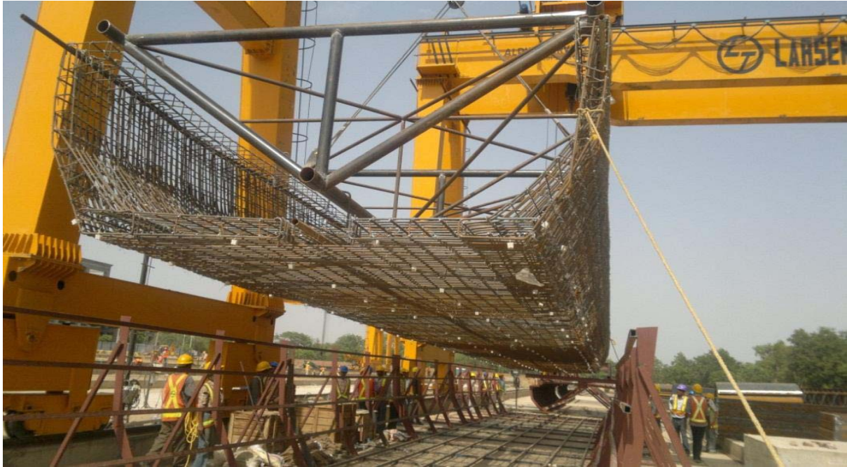
Figure 3.10 Preparation of Reinforcement Cage
