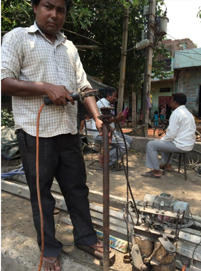
Fig3.10: welding of sprockets on modal steel pile
