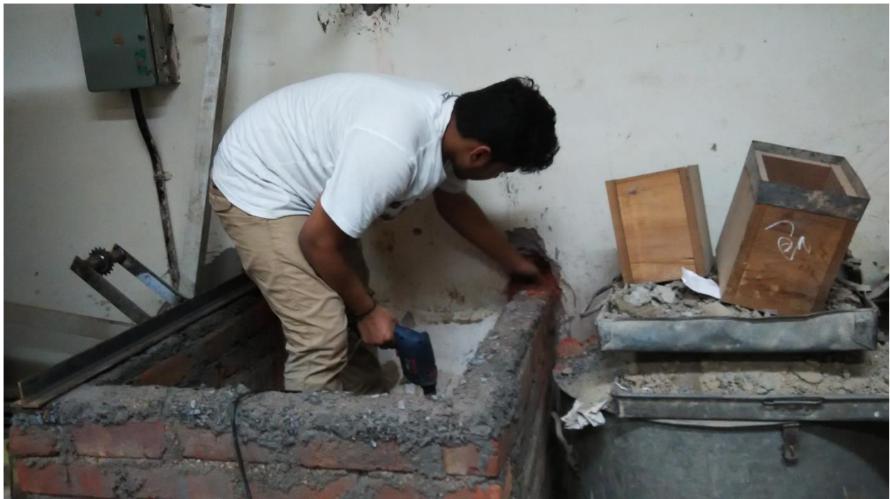
Fig3.5: myself drilling hole in wall to insert a part of girder
