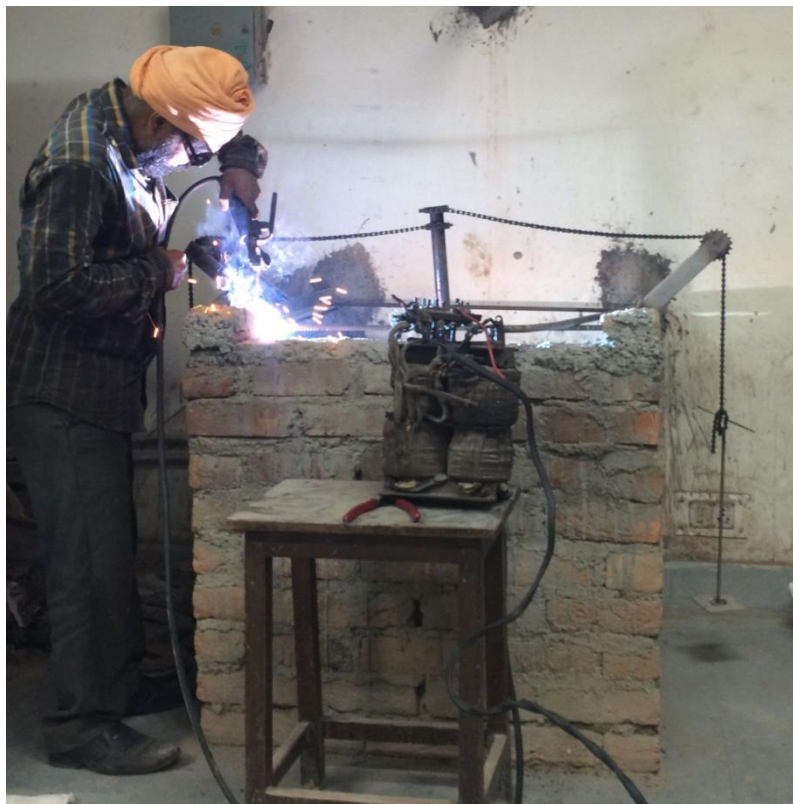
Fig3.12: fixing girders together with steel rods
