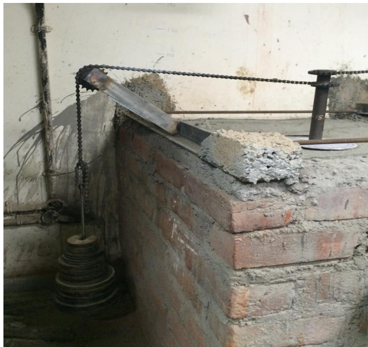
Fig3.7: chain in high tension carrying heavy load to apply torque on pile
