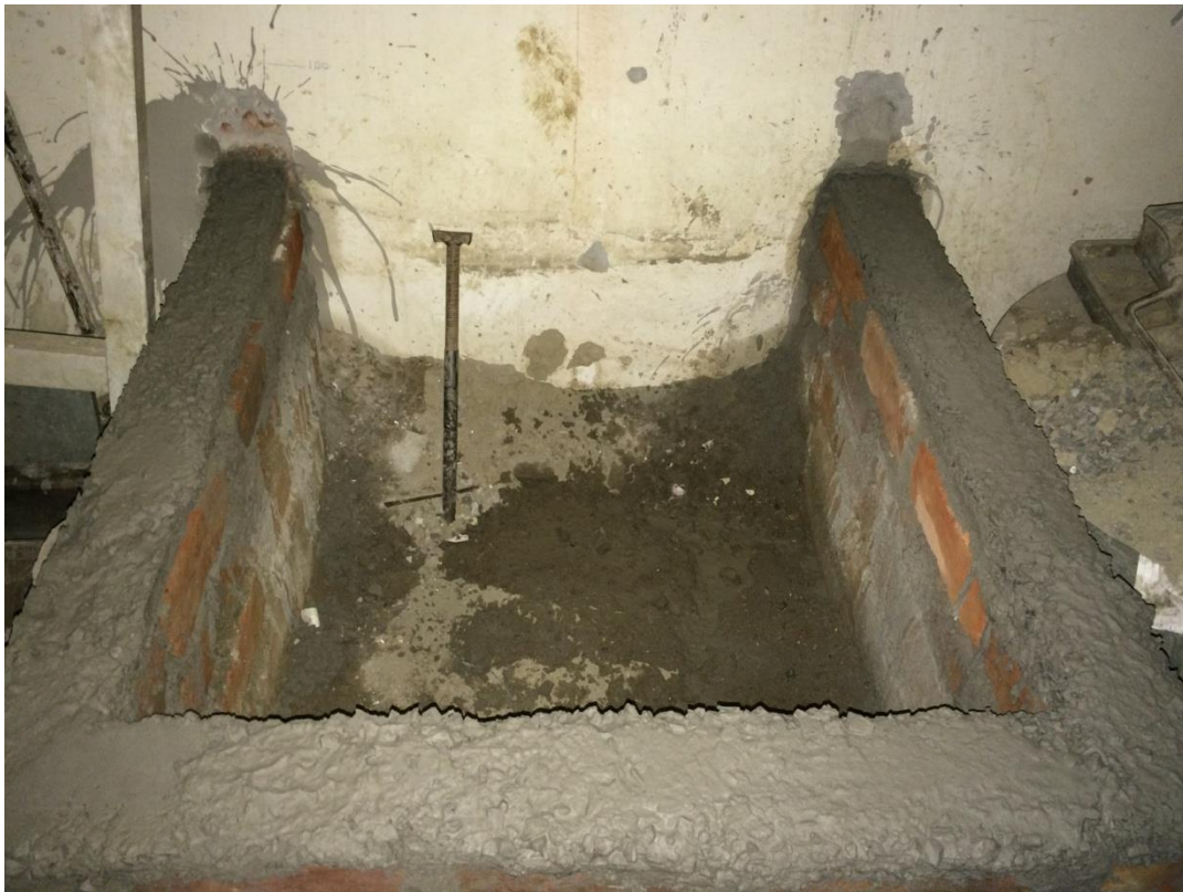
Fig 3.2: Yamuna sand in brick made pit
