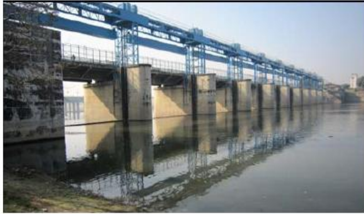
Fig 1.3 Showing Gomti barrage at downstream of Lucknow
