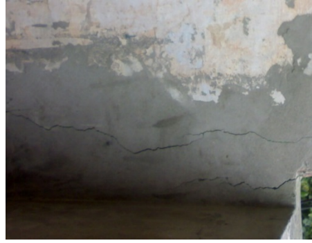
MINOR - DETERIORATION OF PLASTERING
