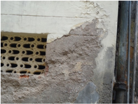
MEDIUM - DETERIORATION OF PLASTERING
