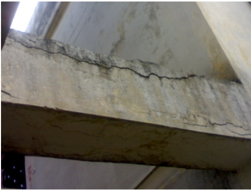
MEDIUM DETERIORATION OF RCC BEAM
