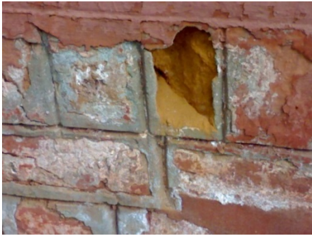
MINOR - DETERIORATION OF BRICK MASONRY
