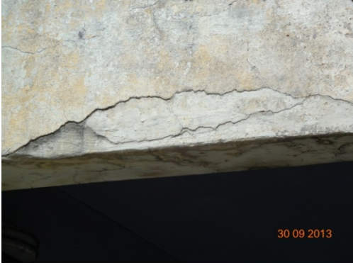
MINOR DETERIORATION OF RCC BEAM
