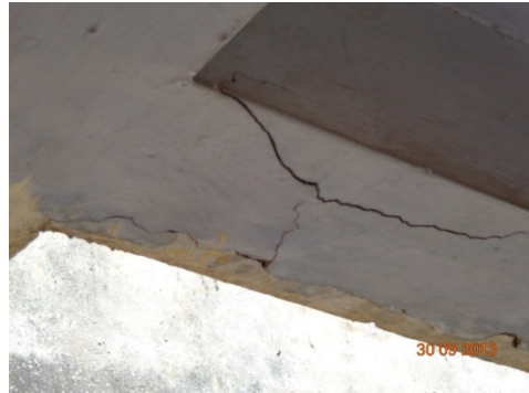
MEDIUM DETERIORATION OF RCC BEAM
