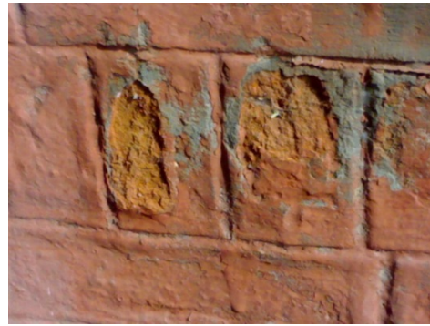
MINOR - DETERIORATION OF BRICK MASONRY
