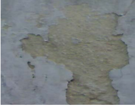
MINOR - DETERIORATION OF PLASTERING
