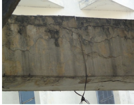
MINOR DETERIORATION OF RCC BEAM
