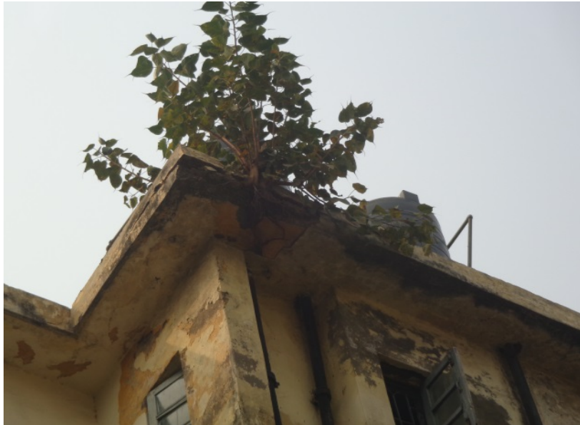
Fig. - 4.1 Vegetation on roof slab
