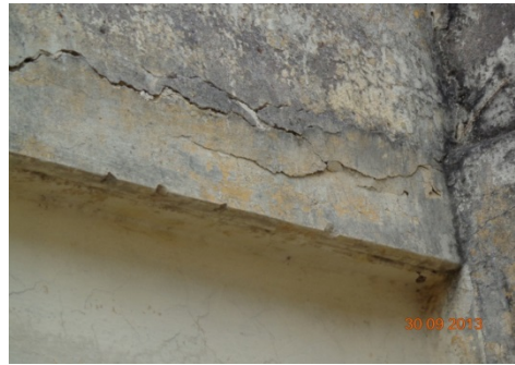
MEDIUM - DETERIORATION OF PLASTERING
