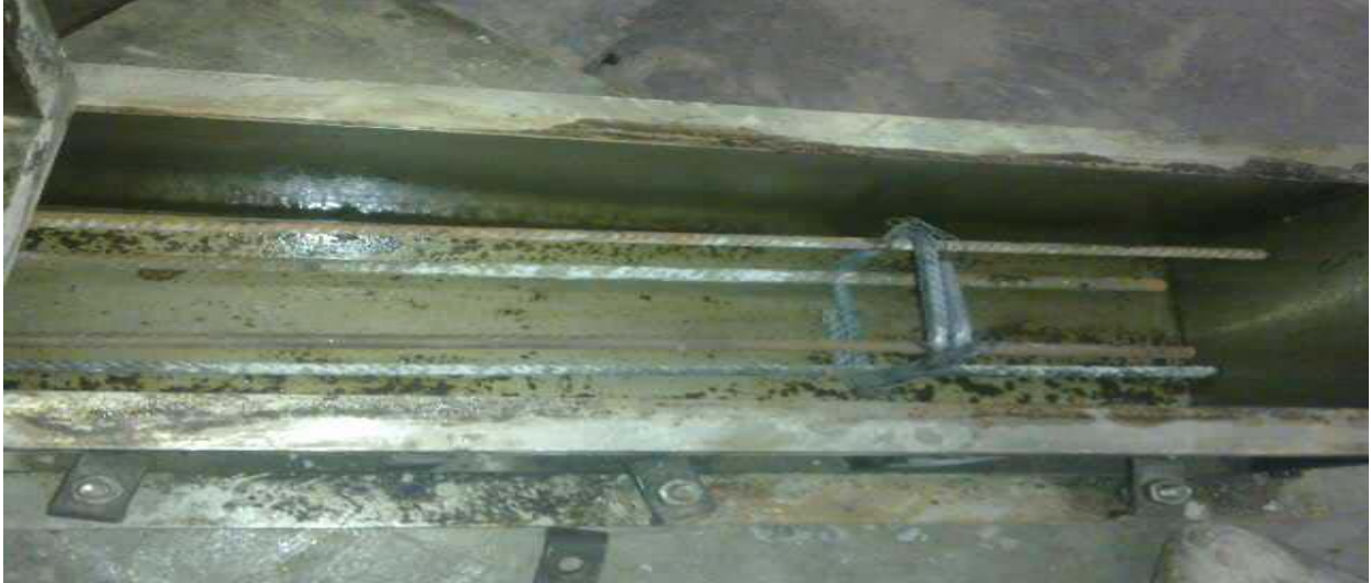
figure 2 .Placement of rings and main bars in beam.
