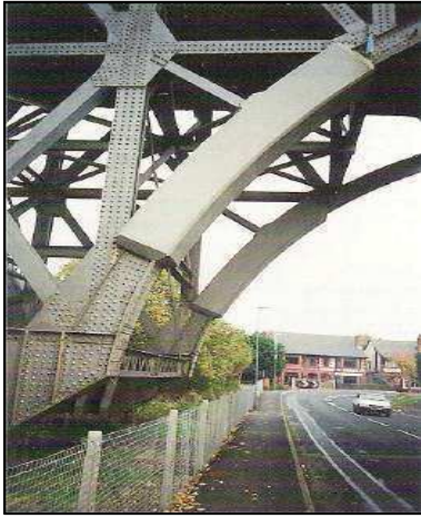
Figure 1: Concrete Covering Retrofit [4]
