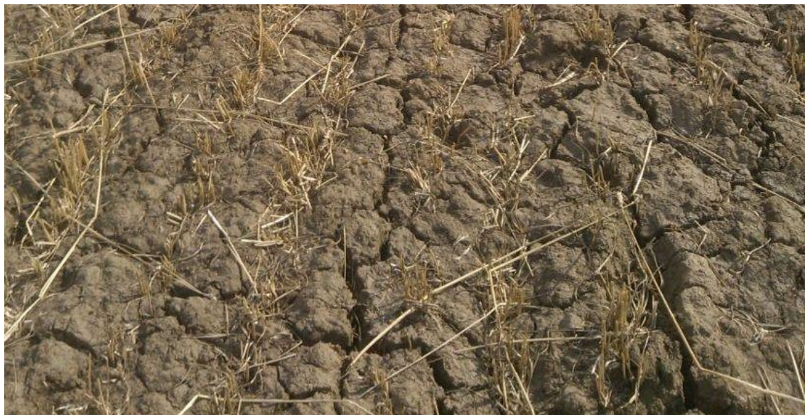
Figure 2: Expansive soil at the site
