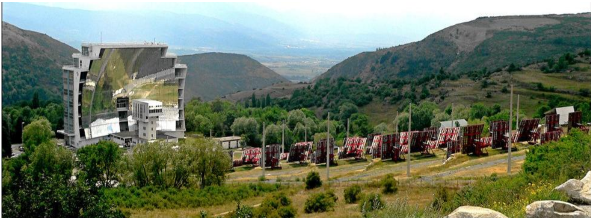
Fig. 2.1 : World's largest solar furnace at Odeillo in France
