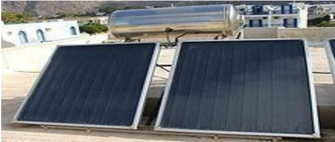
Figure 1.3 Flat-Plate Collectors (NISE) [3]
