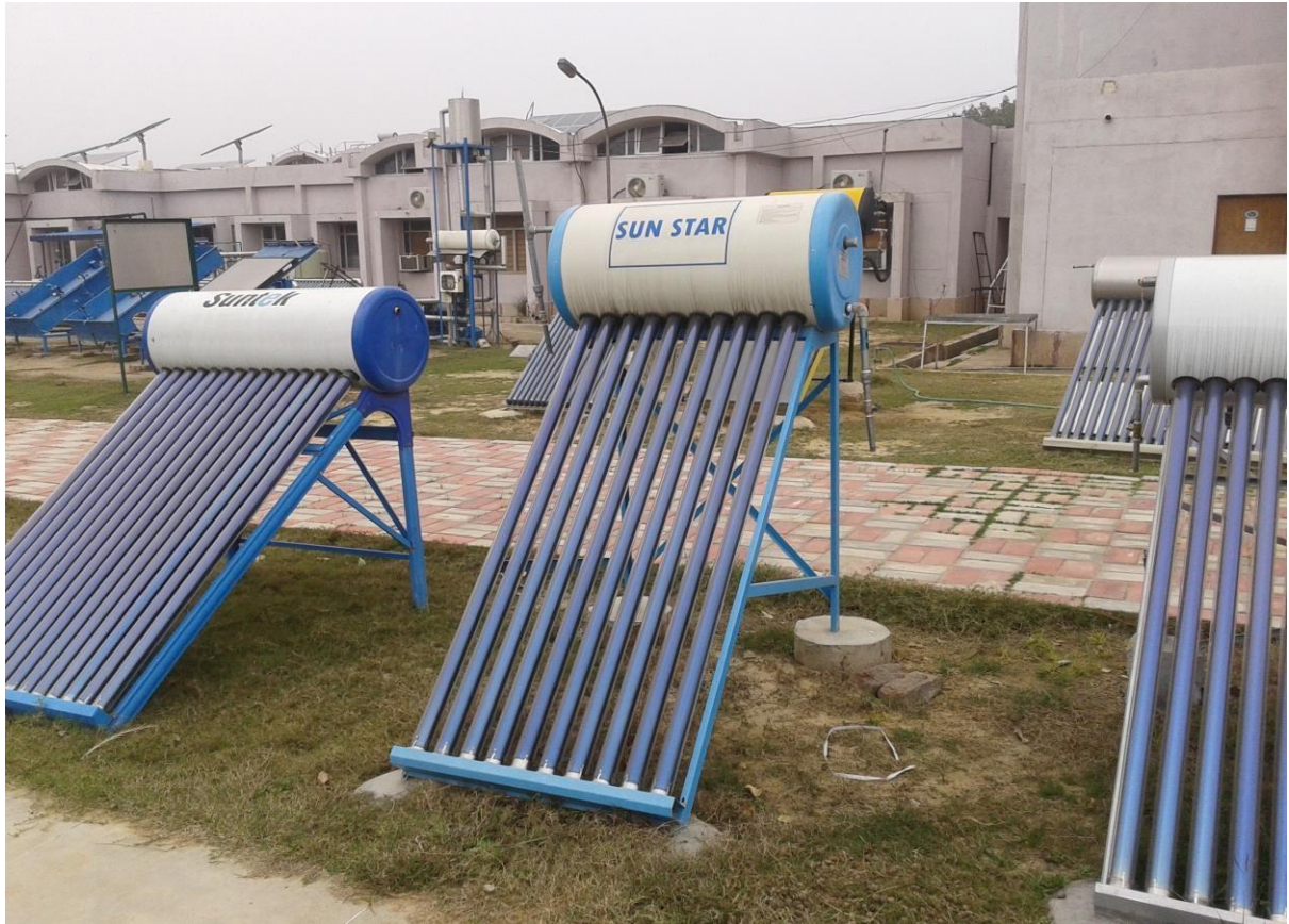
Figure 1.4 Evacuated Tubular Collectors (NISE) [4]
