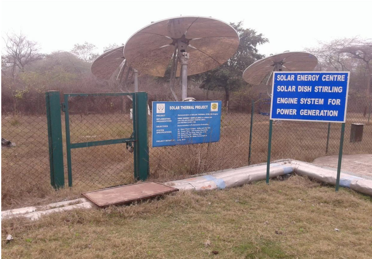
[Figure-1.6 Parabolic Dish collectors (NISE)]
