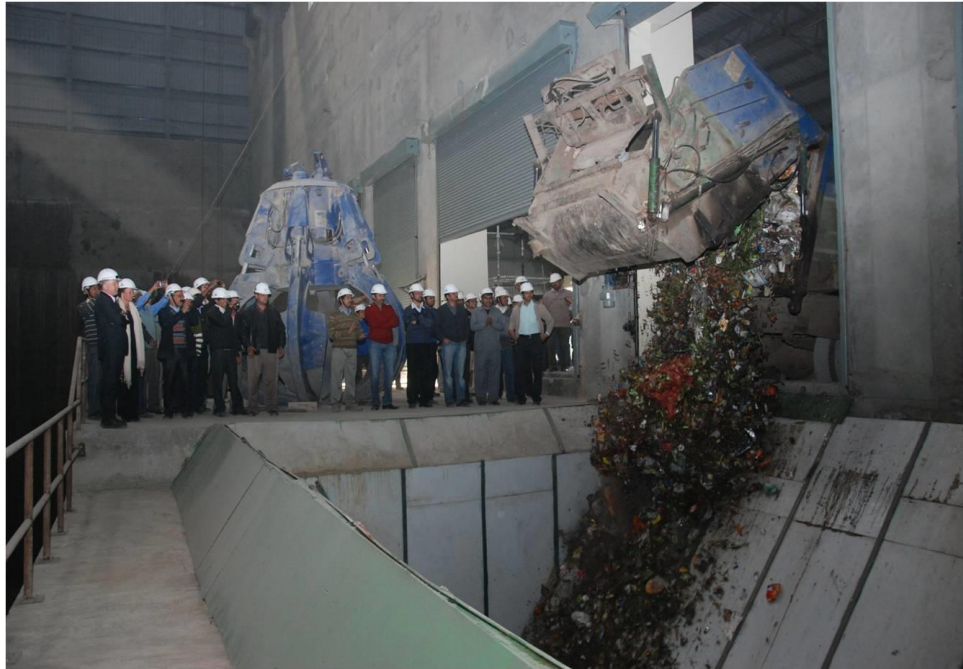
Fig. 3.9: MSW being unloaded at the facility
