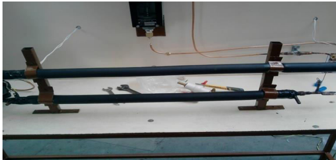
Fig.4.10 Condenser and evaporator
