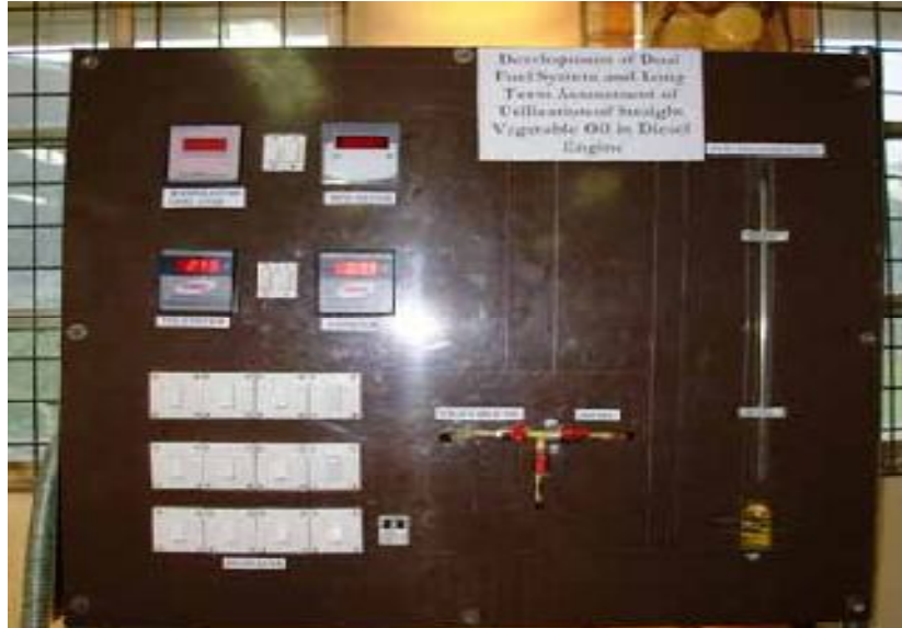
Plate 3.6: Control Panel (front side)
