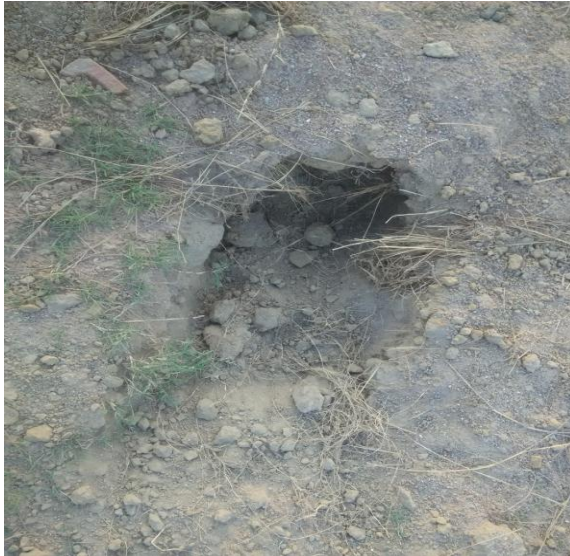
Fig. 3.2(a), Site location.
