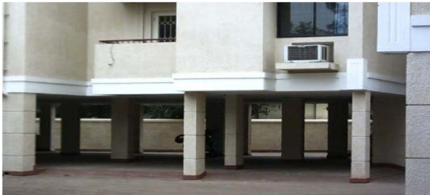
Fig. 1.1: Typical example of OGS building
