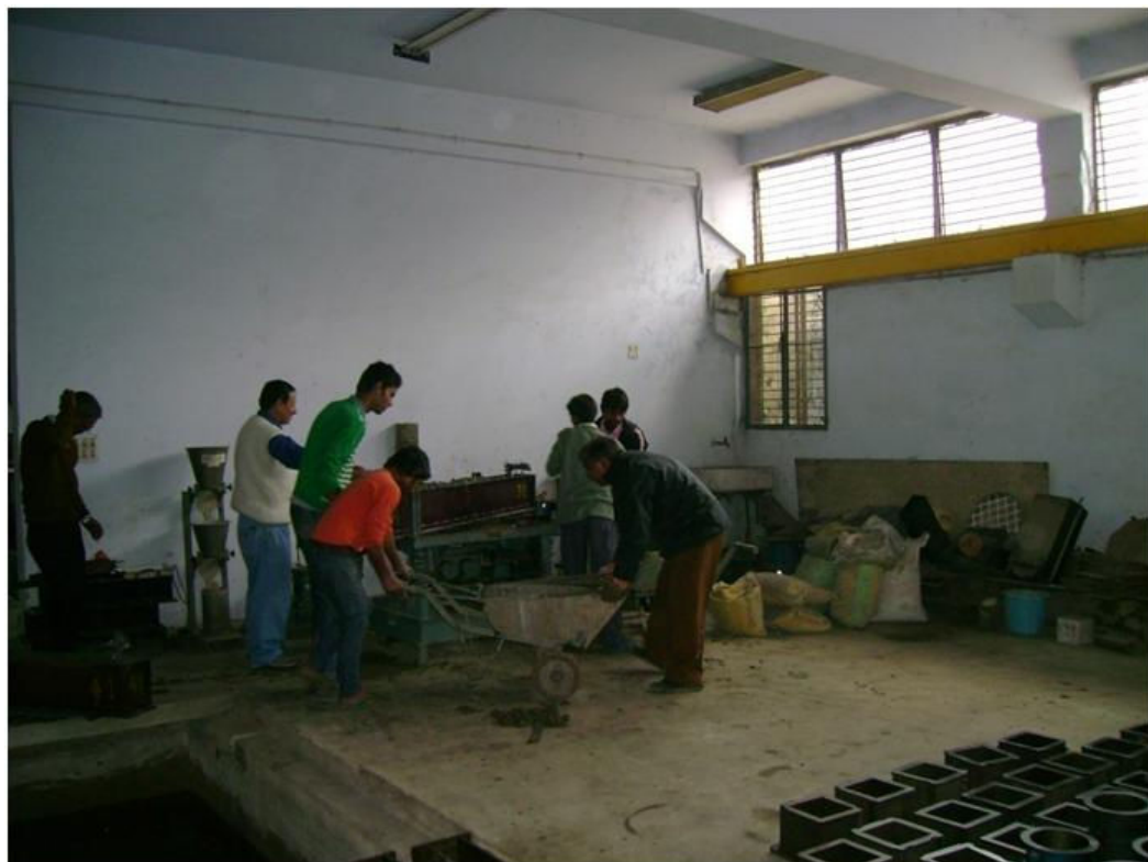
Fig. 38 Casting of Beam on Table Vibrator
