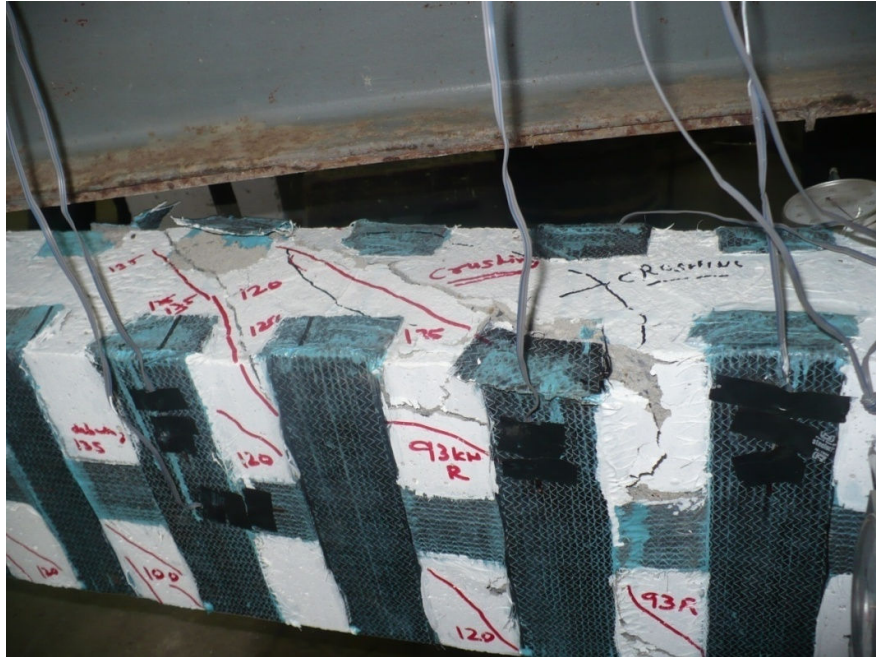
Fig. 87 Top View Failure of Crushing of Concrete
