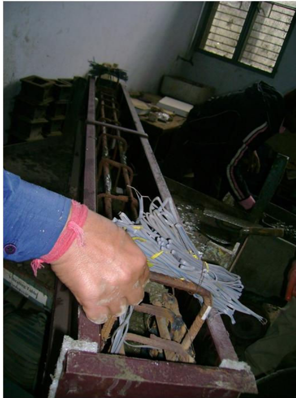
Fig. 39 Protecting the Electric Strain Gauges for Damaging during Concreting
