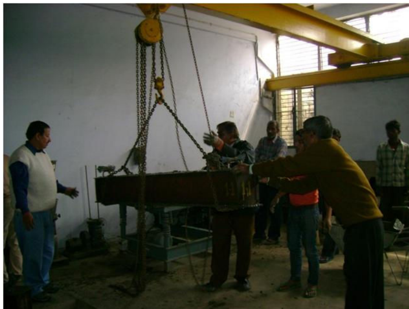
Fig. 40 Lifting of Beams from Table Vibrator after casting
