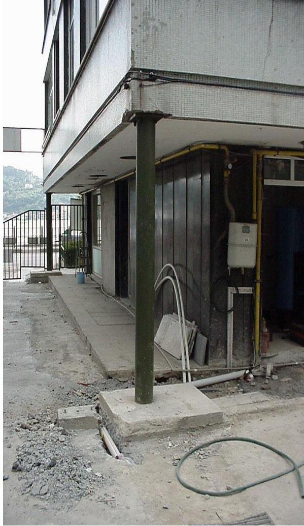
Fig.1.13d) Additional column.
