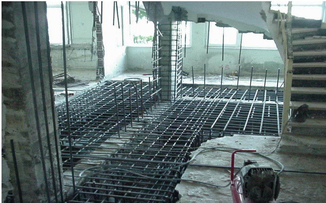
Fig. 1.13a) Additional foundations.
