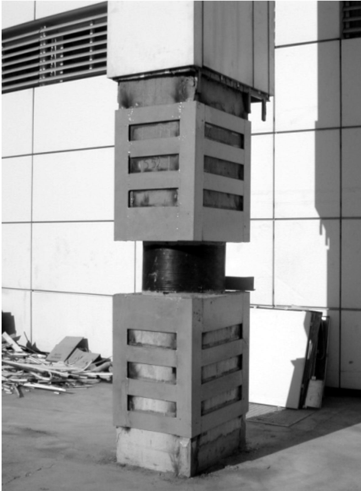
Fig 1.17: Steel jackets replacing the discontinued reinforcing bars.
