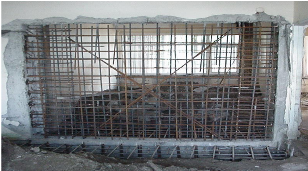
Fig 1.13 b) Additional shear walls.
