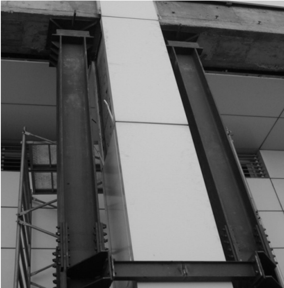
Fig. 1.14 Installation of temporary steel props.
