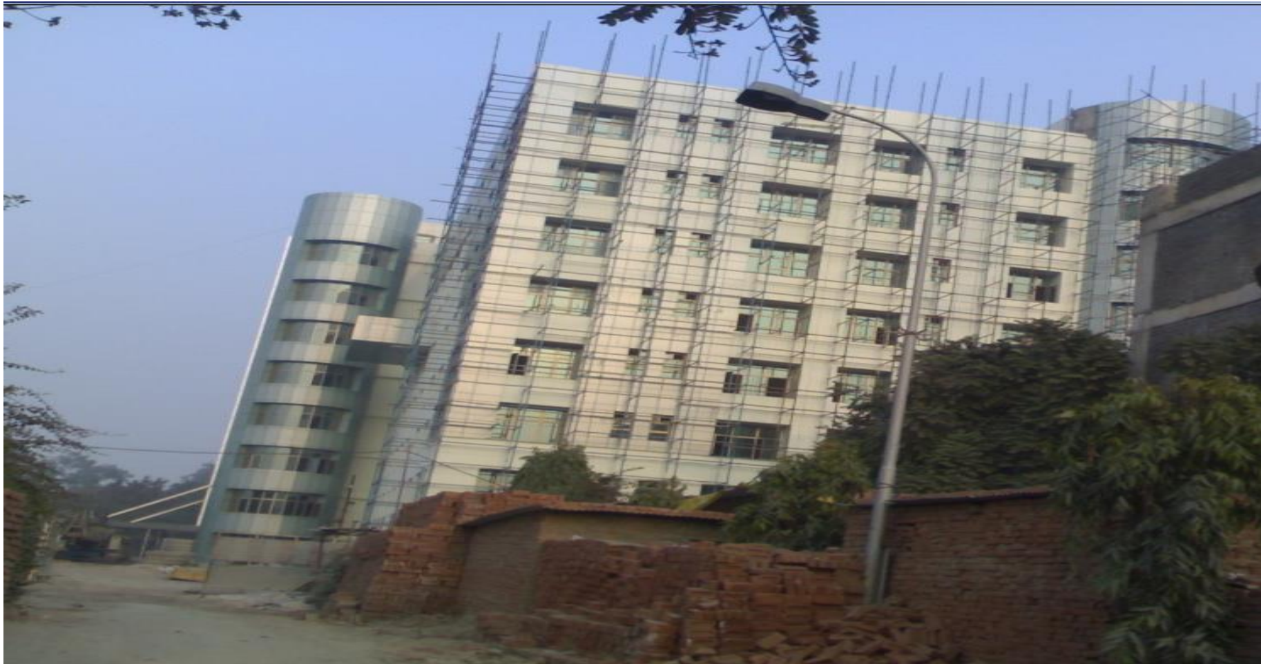
A View of Base-Isolated 9 Storey Building Constructed in the Dilshadgarden GTB Hospital Delhi
