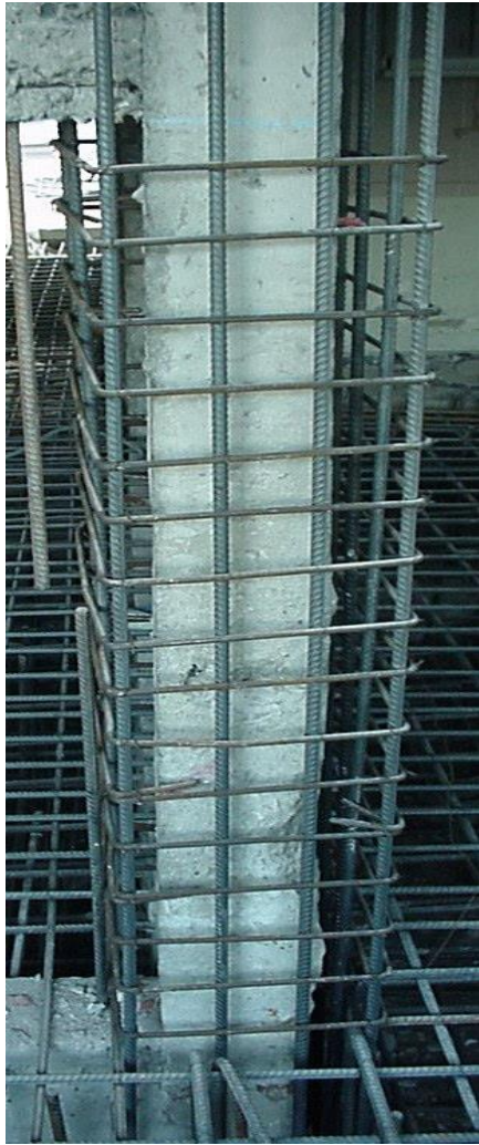
Fig. 1.13c) Jacketing of column.
