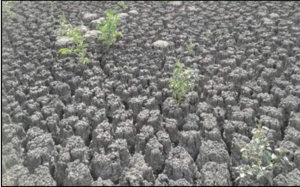
Figure 5.53: Sludge Drying Beds at Oxidation Ditch based STP
