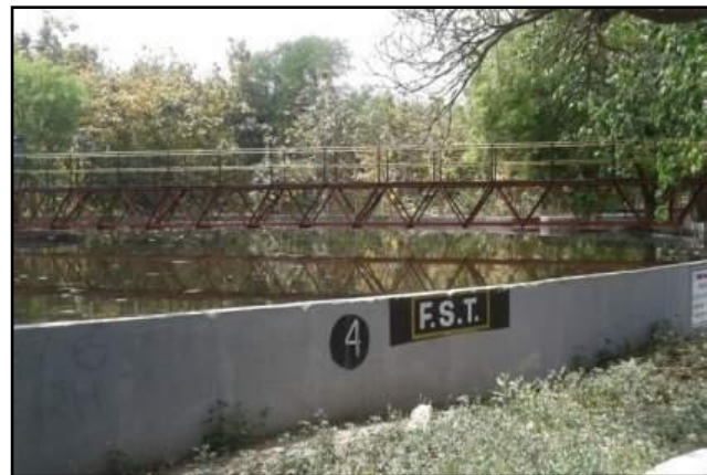
Figure 5.36: Final Settling Tank of ASP Plant
