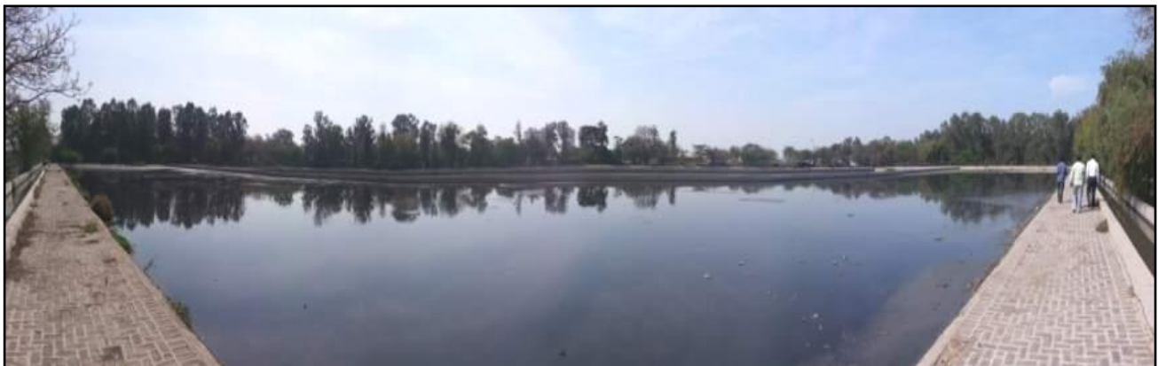
Figure 5.27: Final Polishing Unit after UASB Reactor
