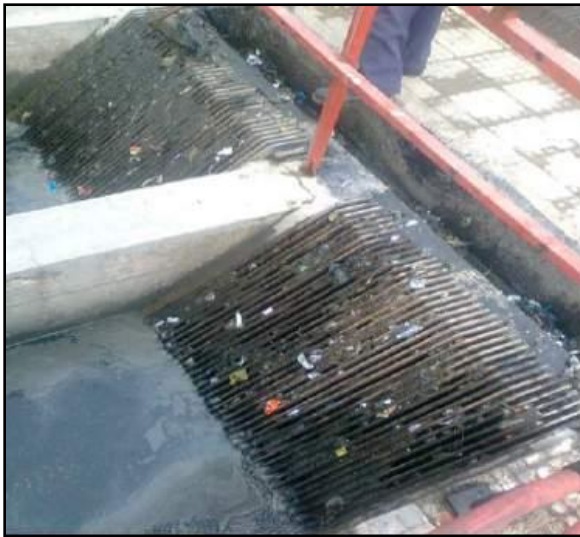
Figure 5.2: Fine Screens in BIOFOR based STP
