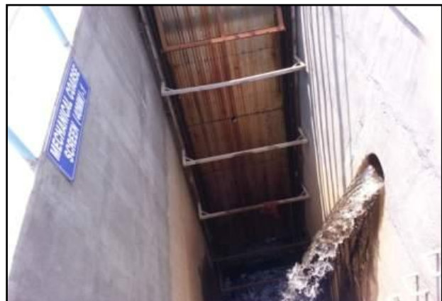
Figure 5.13: Coarse Screen: 40mm at SBR based STP
