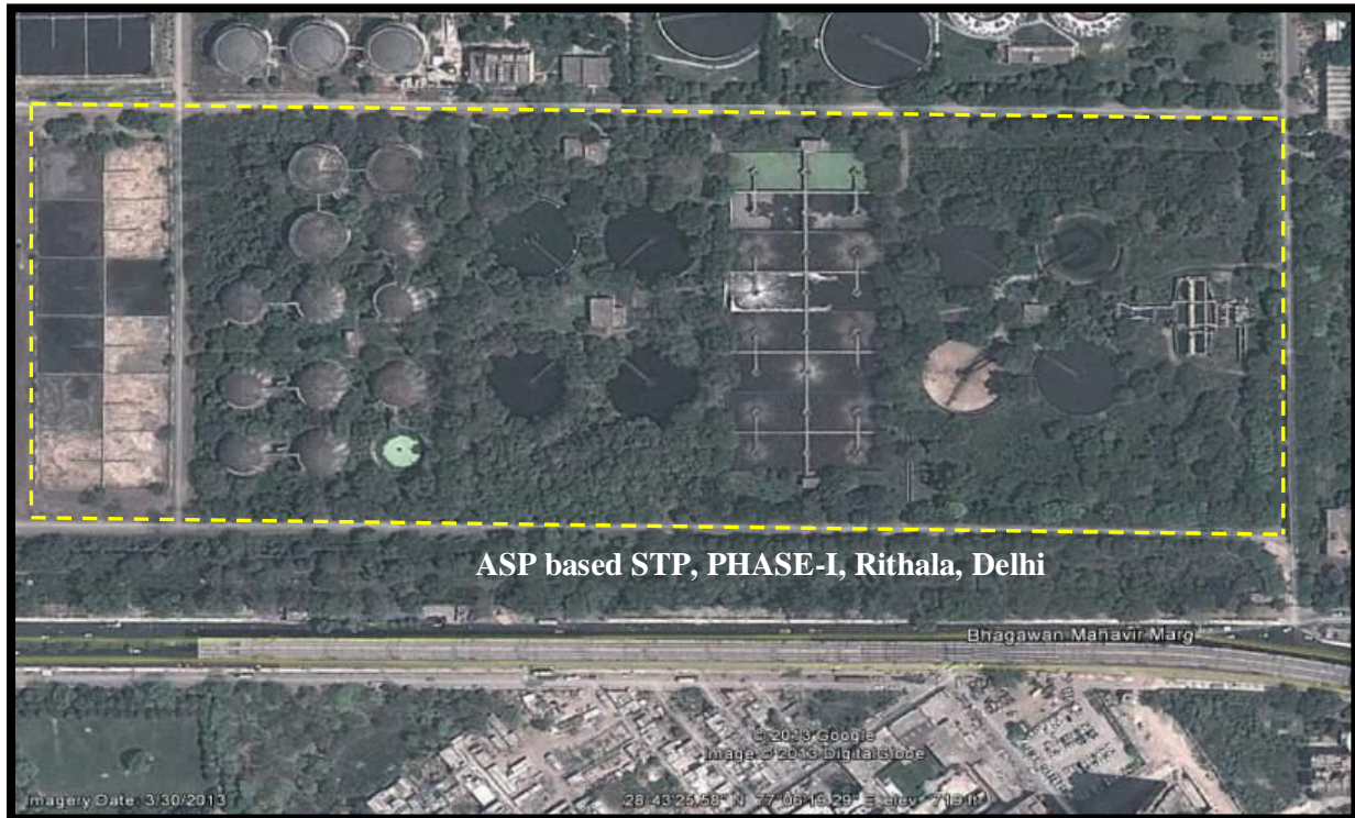
Figure 5.33: Satellite image of STP based on ASP at phase-I, Rithala, Delhi
