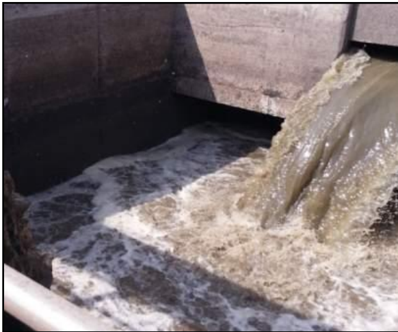
Figure 5.15 Fill Aerate phase of SBR Cycle
