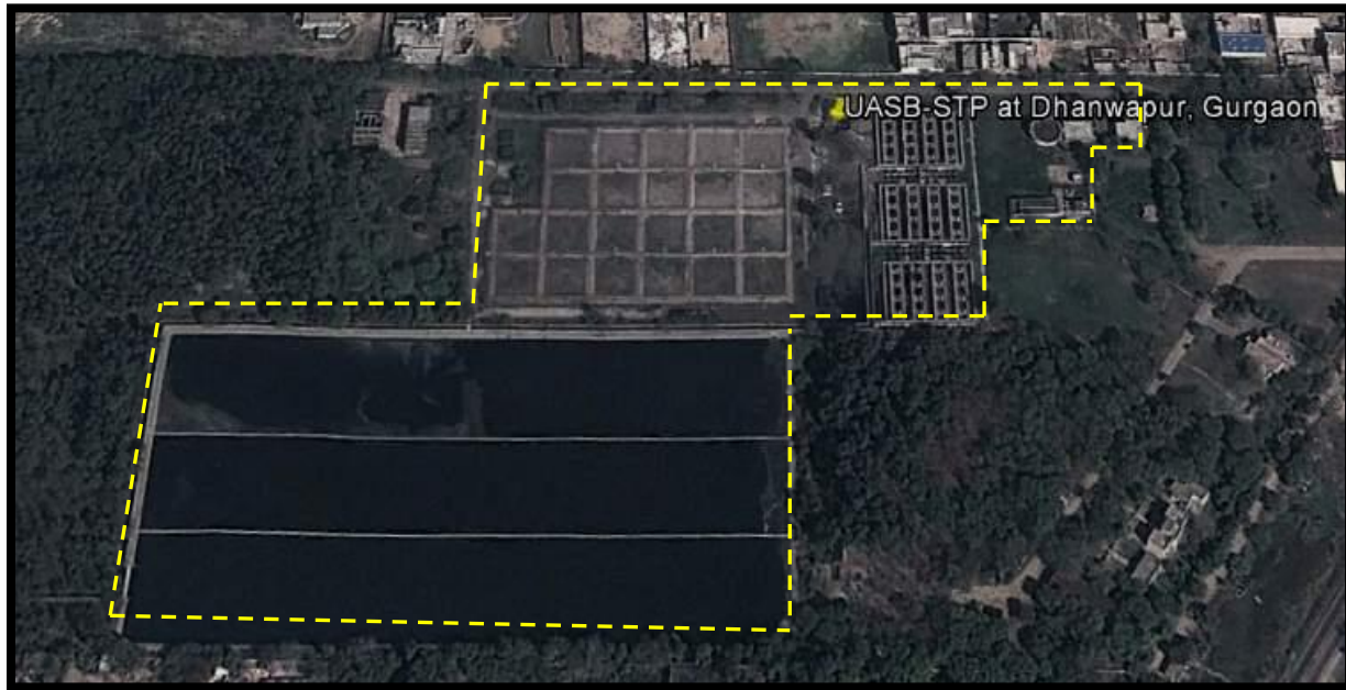
Figure 5.24: Satellite image of STP based on UASB at Dhanwapur, Gurgaon, Haryana
