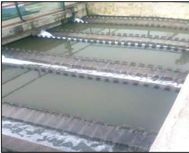
Figure 5.5: BIOFOR Stage – I Filtration
