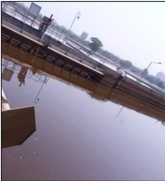
Figure 5.17: Settle Phase of SBR Cycle
