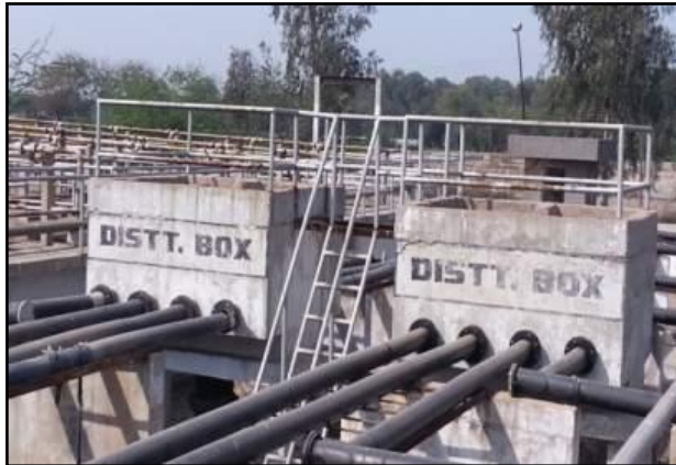
Figure 5.25: Distribution Chambers for UASB reactor
