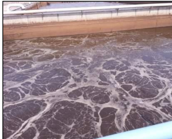
Figure 5.16 React phase of SBR Cycle
