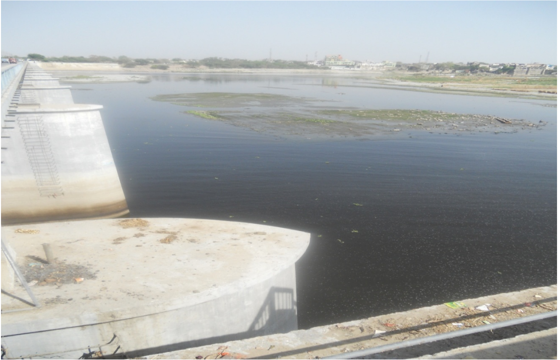
Fig 5.20: Downstream of Gokul Barrage
