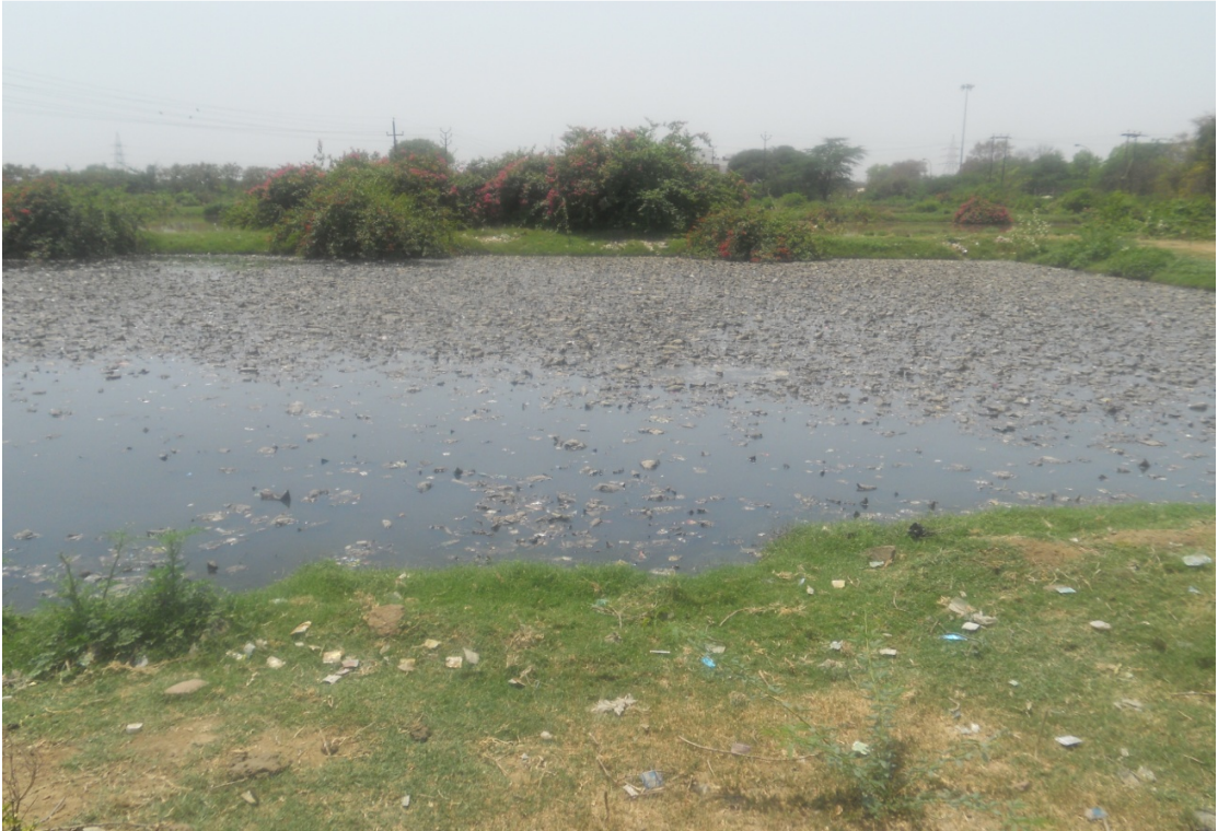
5.16: Oxidation pond at Pagalbaba STP
