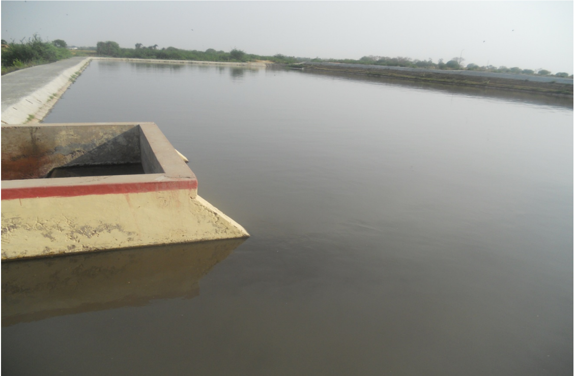
Fig 5.31: Oxidation pond at Pilakher STP
