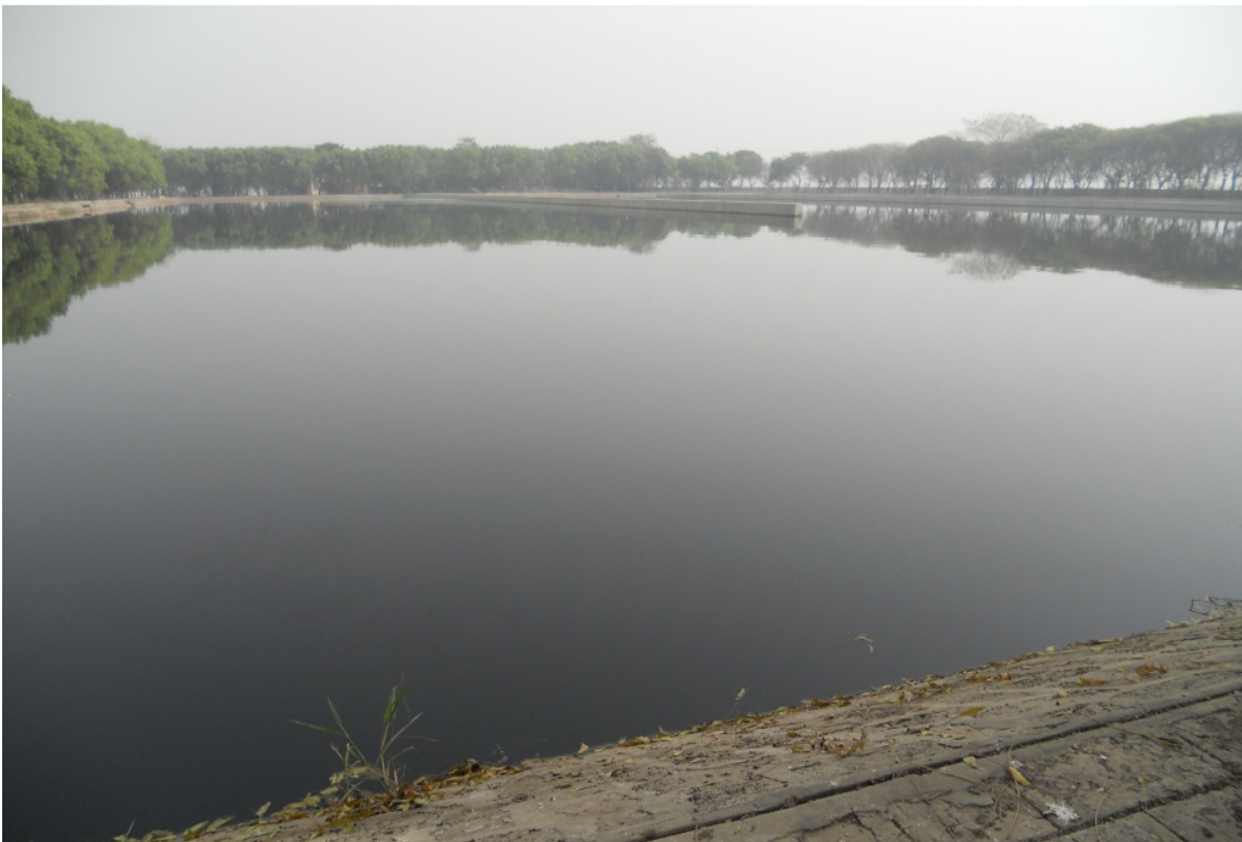
Fig 5.11: Oxidation Pond of Faridabad STP
