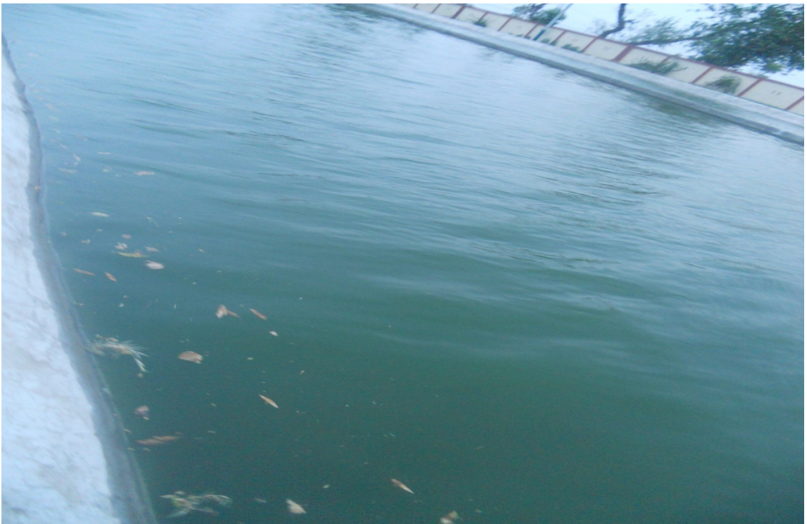
Fig 5.33: UASB and Oxidation pond at Bhimnagri STP.
