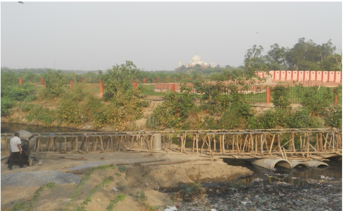
Fig 5.28: Red fort drain.
