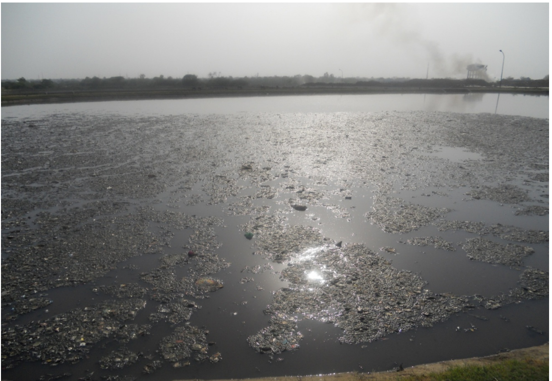
Fig 5.21A: Oxidation pond of Trans-Yamuna STP, Mathura
