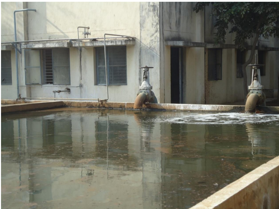
Fig 4.4: Pre-chlorination tank
