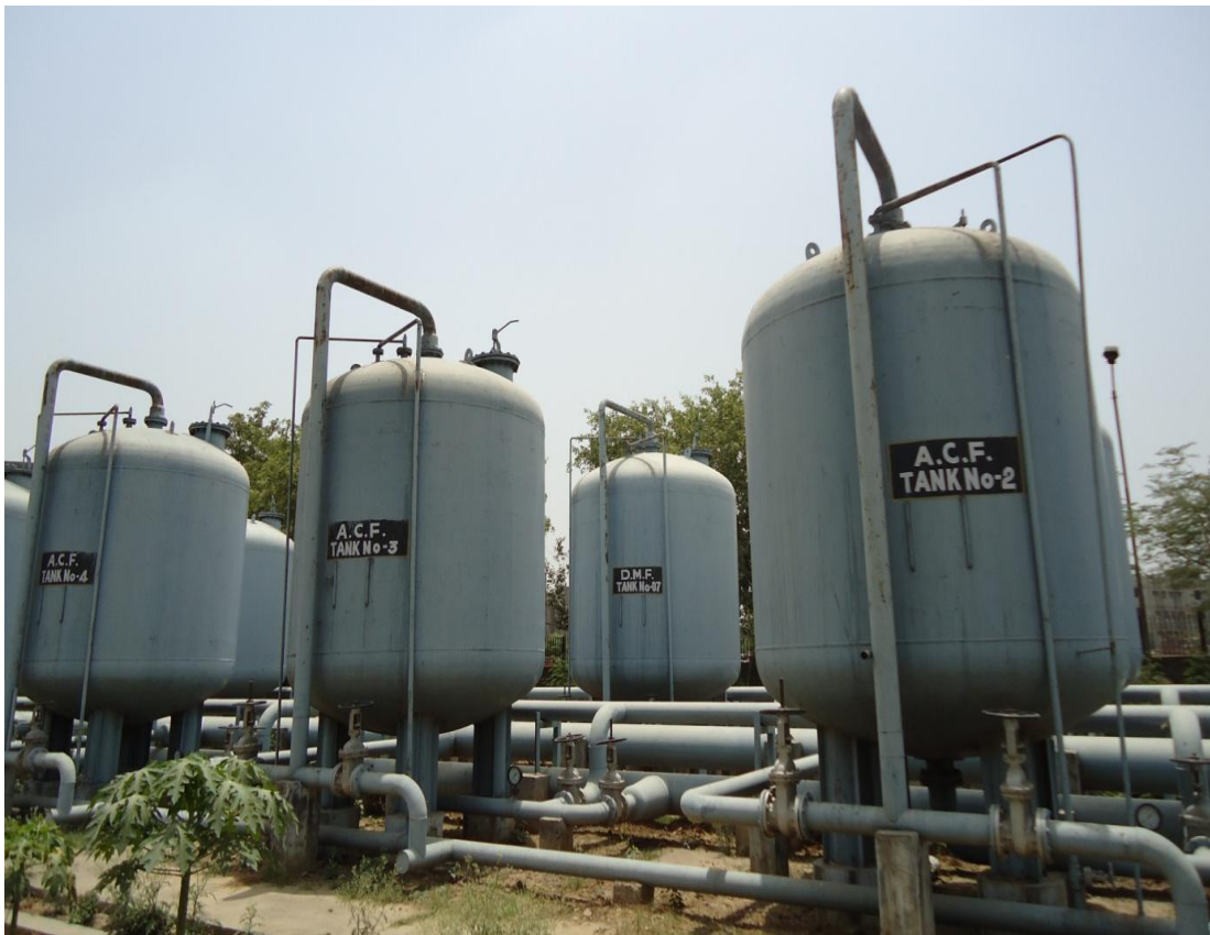
Fig 4.8: Activated Carbon filter
