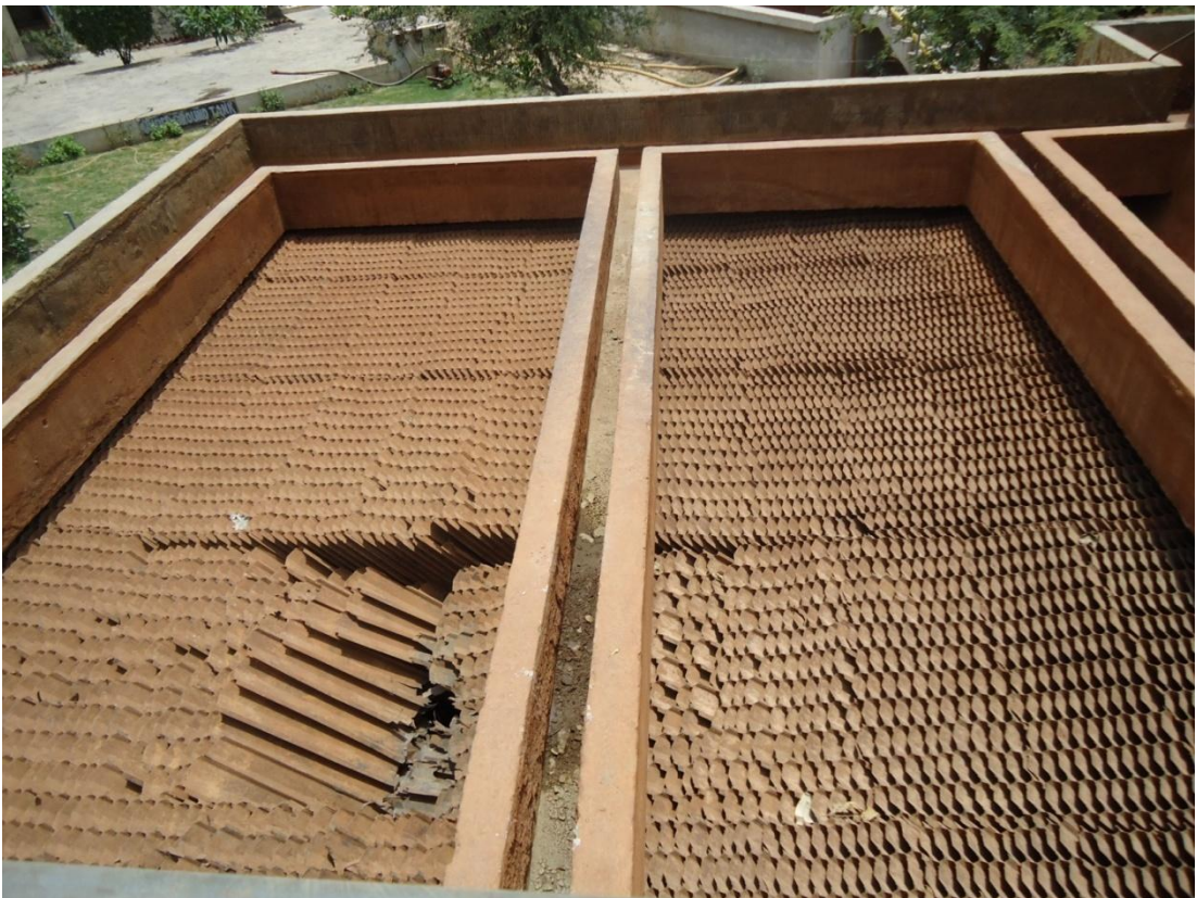
Fig 4.6: Tube Settler
