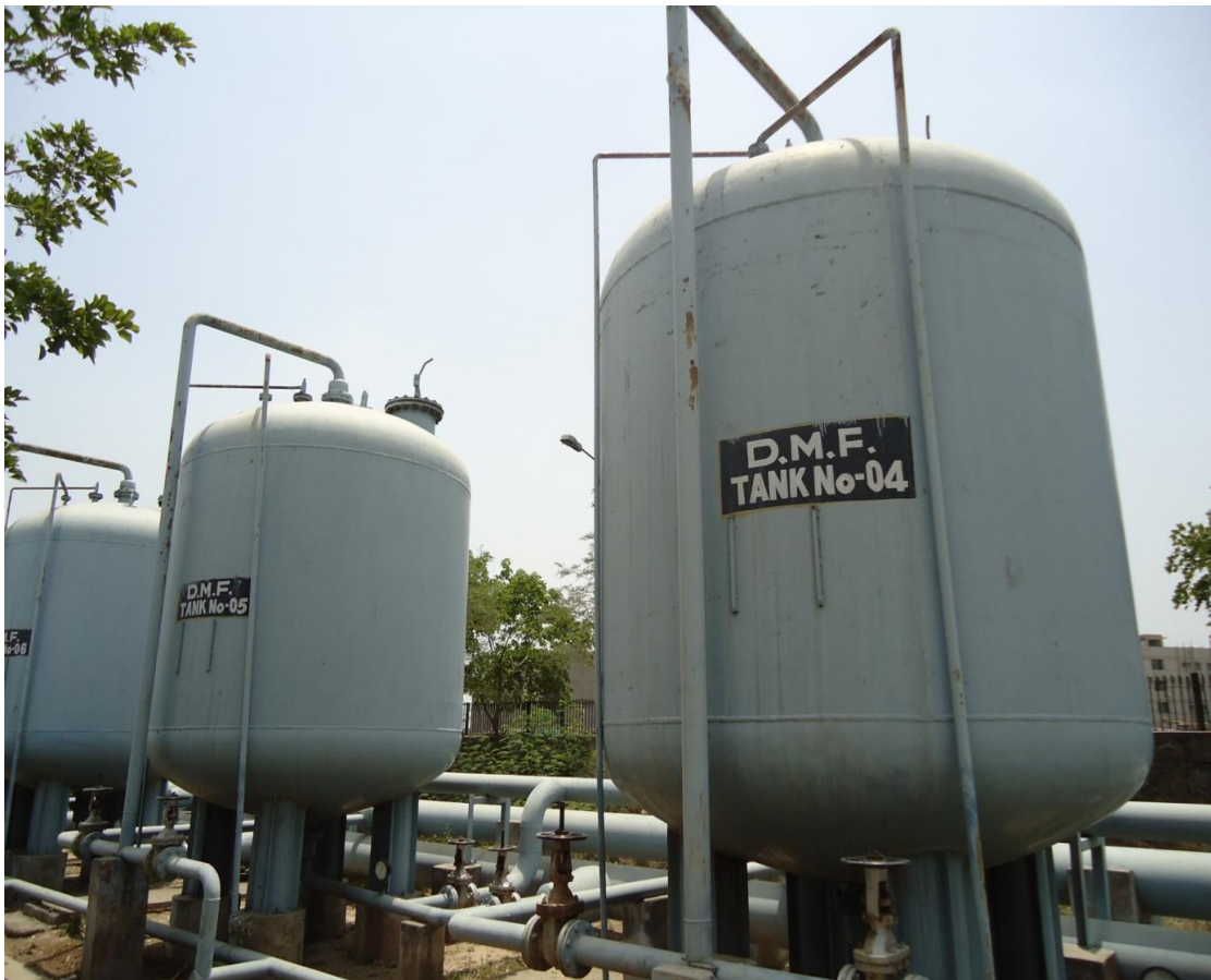
Fig 4.7: Dual Media Filter
