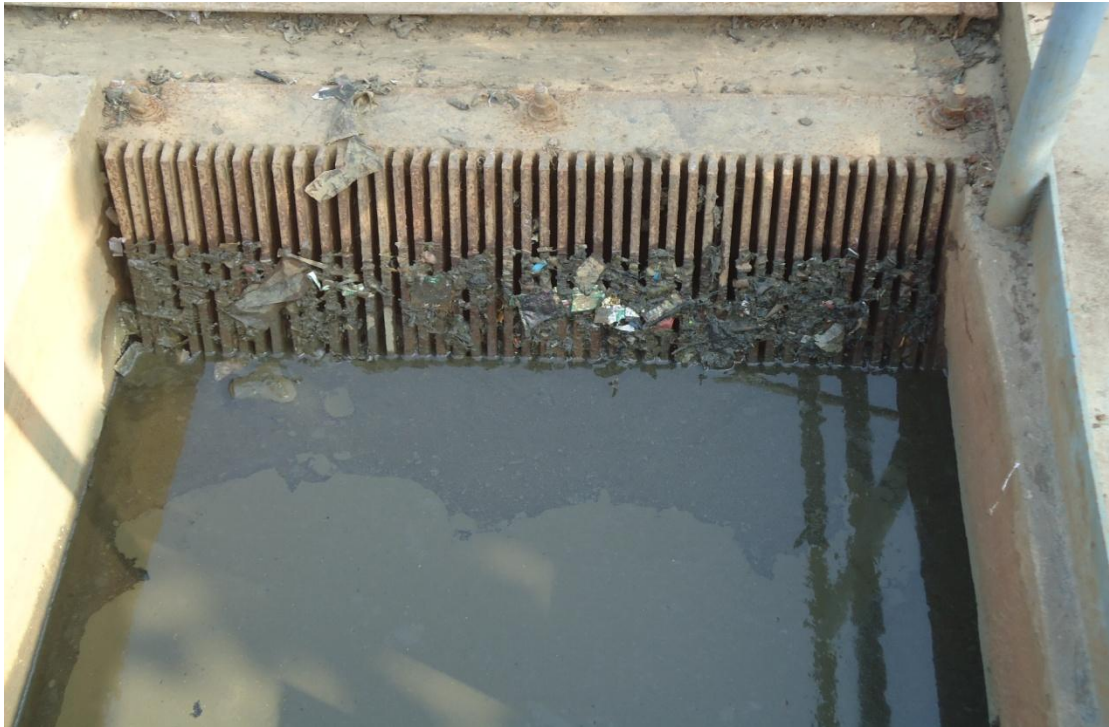
Fig 4.1: Screen chamber
