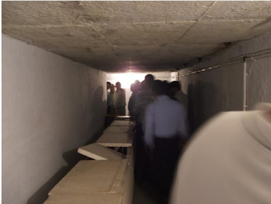
Fig.3.28: Basement of the Seismological Laboratory
