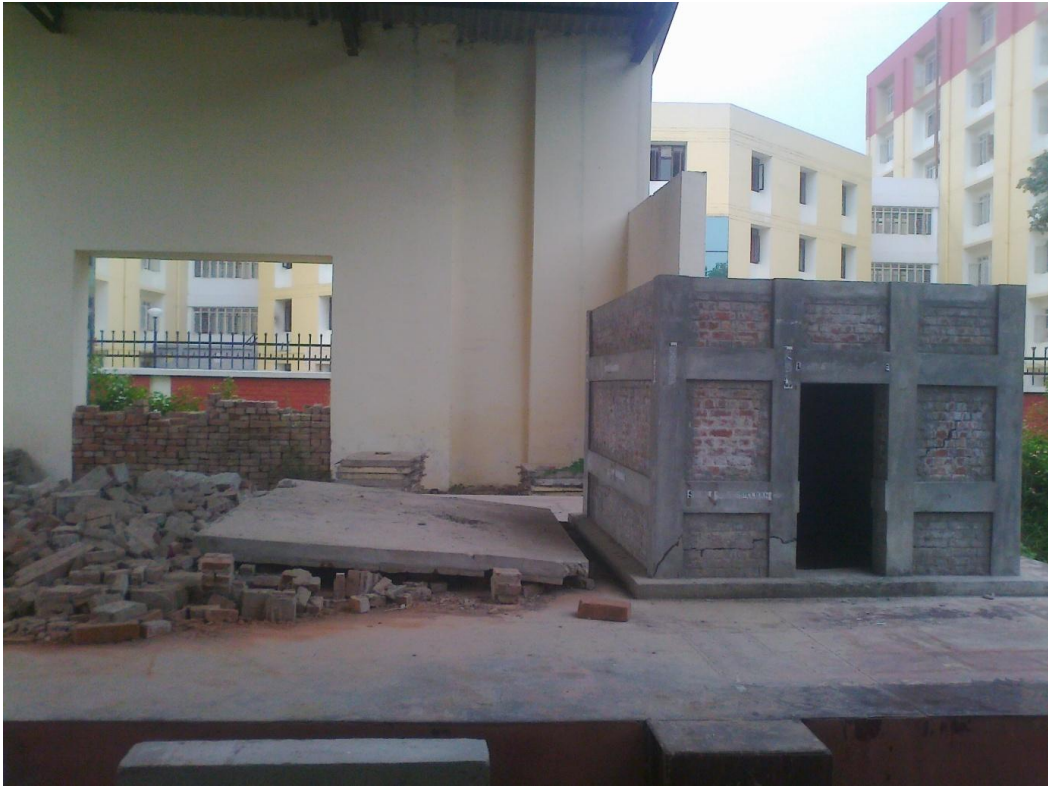
Fig.3.12: Behaviour of the normal reinforced building and earthquake resistant brick masonry building due to lateral shock
