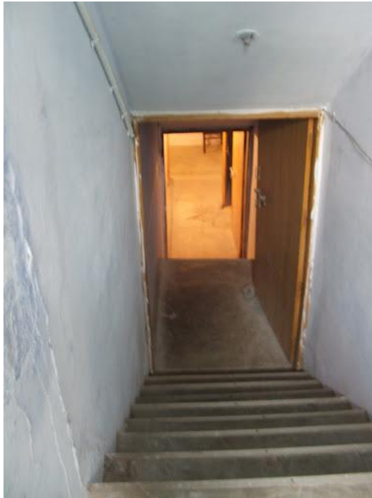
Fig.3.27: Way to the Basement of the Seismological Laboratory
