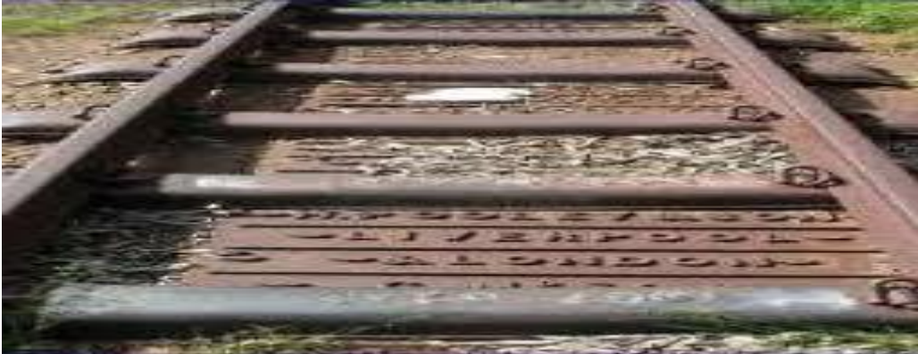
Fig 3.3- Cast Iron Sleepers
