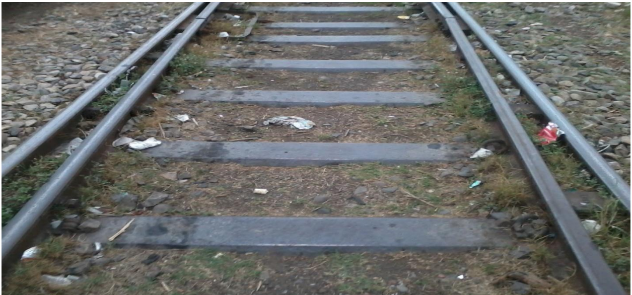
Fig 3.2- Steel Through sleeper
