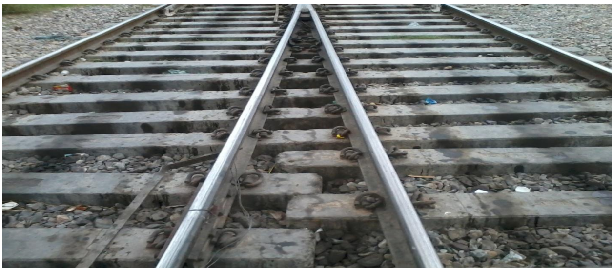
Fig3.6 -PRC sleepers for turn outs
