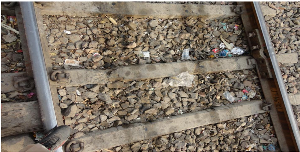
Fig4.2- Bending cracks
