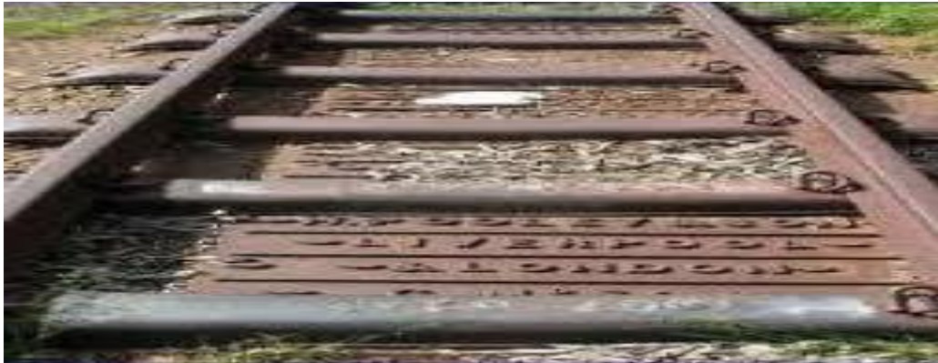
Fig 3.3- Cast Iron Sleepers
