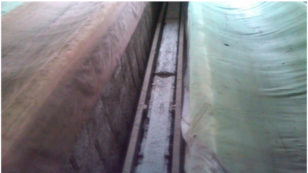
Fig 5.6 Steam curing
