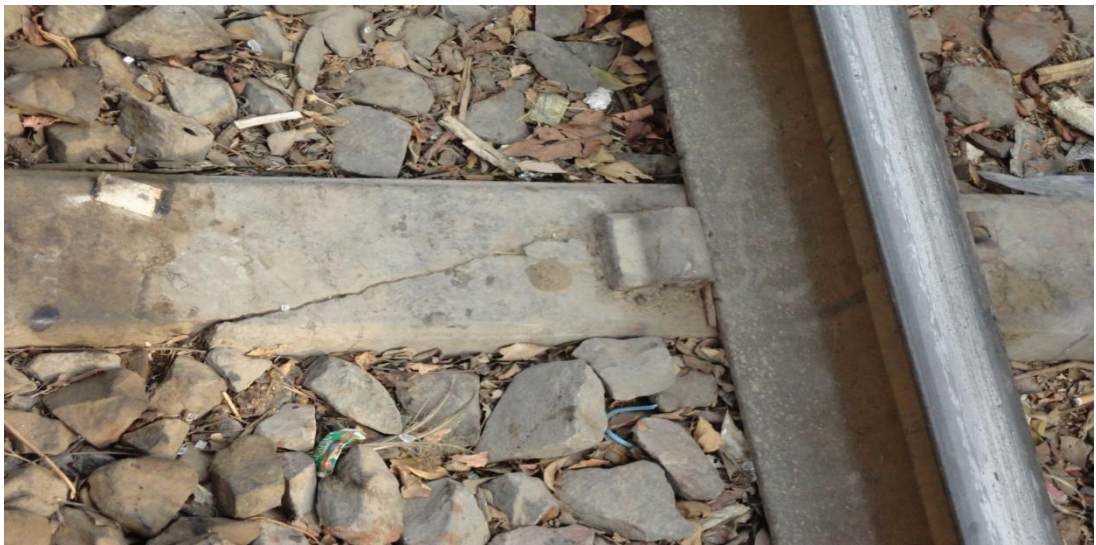
Fig4.4- Cutting Cracks
