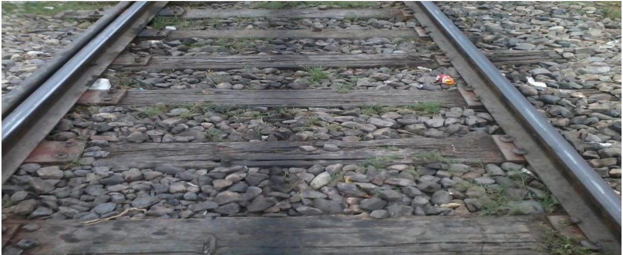
Fig 3.1- Wooden Sleepers
