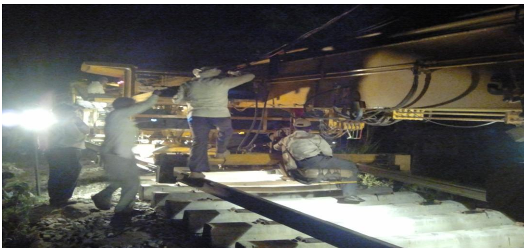
Fig 6.2 Track Relaying Train
