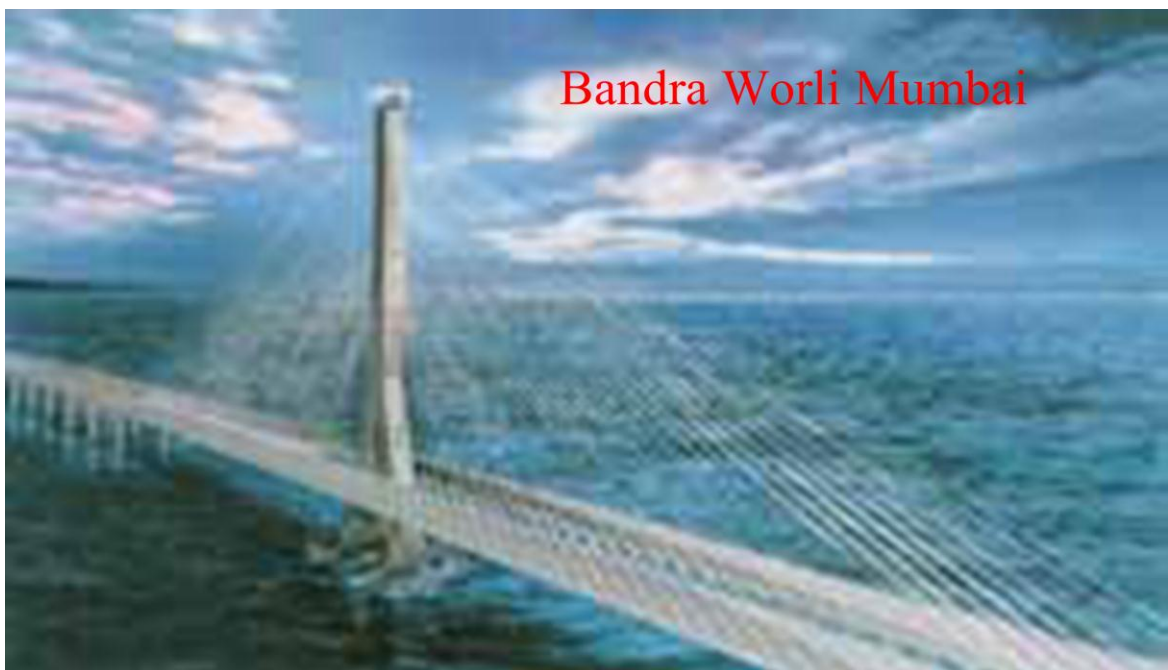
Fig.2.4 Bandra worli bridge, mumbai(source- Elkem microsilica)
