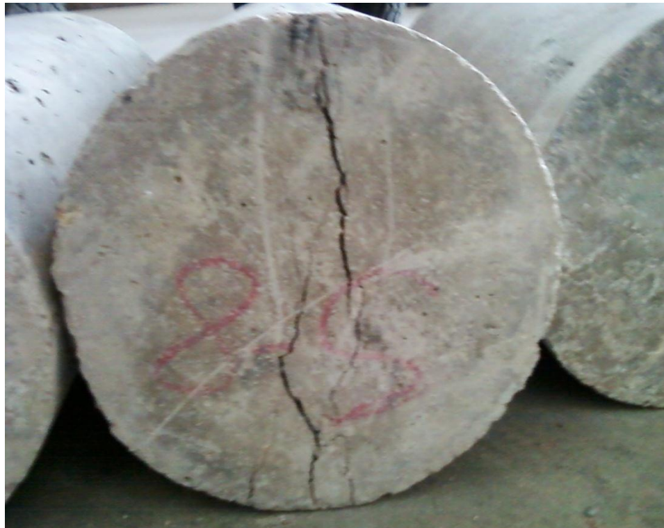
Fig.3.3 Specimen failed in tension (vertical crack is appeared)
