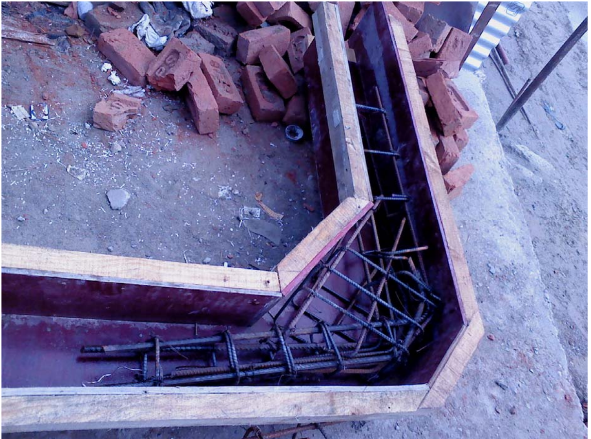
Figure 65: Specimen C before casting
