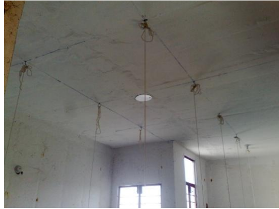
Fig 3 Showing plumb bobs suspending from the roof
