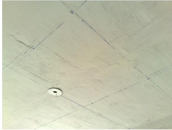
Fig.1 Showing marking on roof slab
