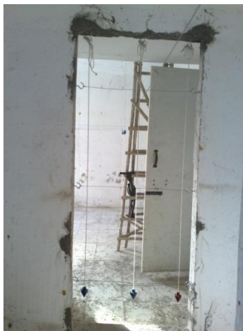
Fig.2 Door opening created in casted wall
